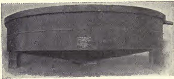
FIG. 123.—Steel Tank, 70 ft. diam., for Rand Practice.
