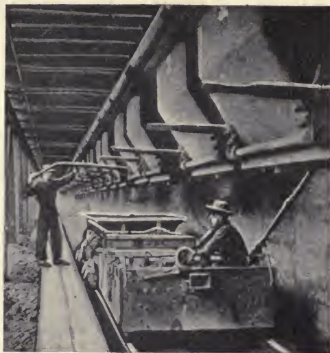
FIG. 253.—Charging Feed-car.
