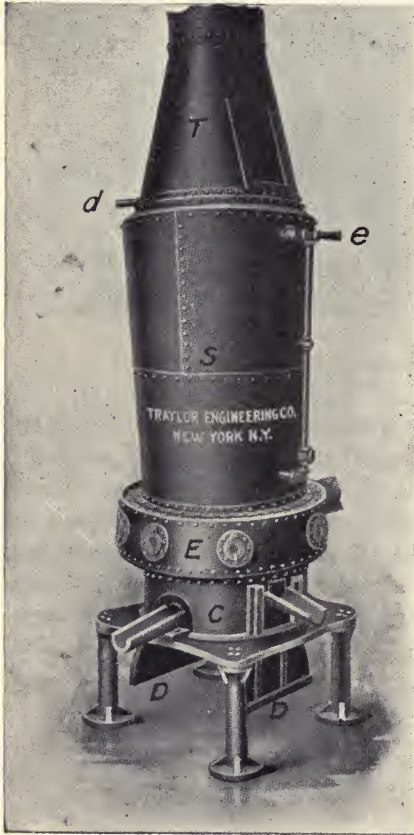
FIG. 62.—Cupola Blast Furnace.
