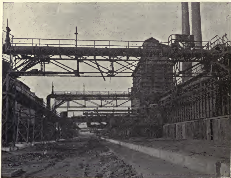
FIG. 12.—Perspective View, Ovens, Coke-pusher and Leveler.
