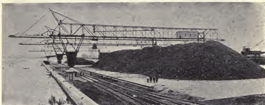
Fig. 151.—Three Traversing-bridge Tramways with 5½-ton Grab-buckets; Storage capacity, 500,000 tons.
