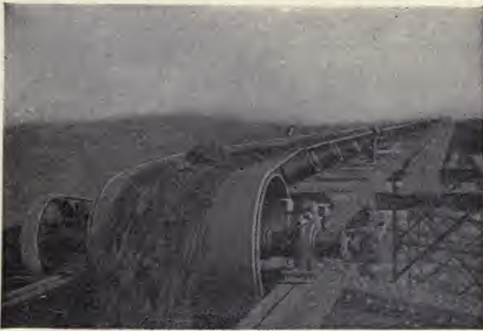
FIG. 314.—Discharge at Head of Conveyor.
