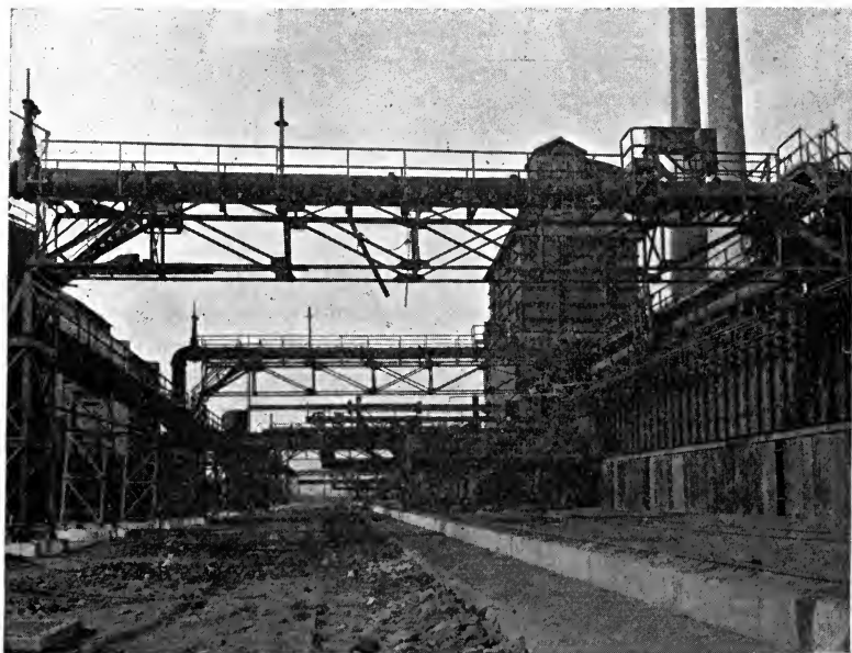
FIG. 12.—Perspective View, Ovens, Coke-pusher and Leveler.
