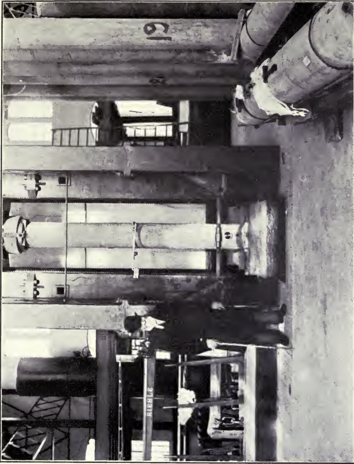
FIG. 15.—THE FRITZ ENGINEERING LABORATORY, INTERIOR. 800,000 POUND RIBBLE TESTING MACHINE.
