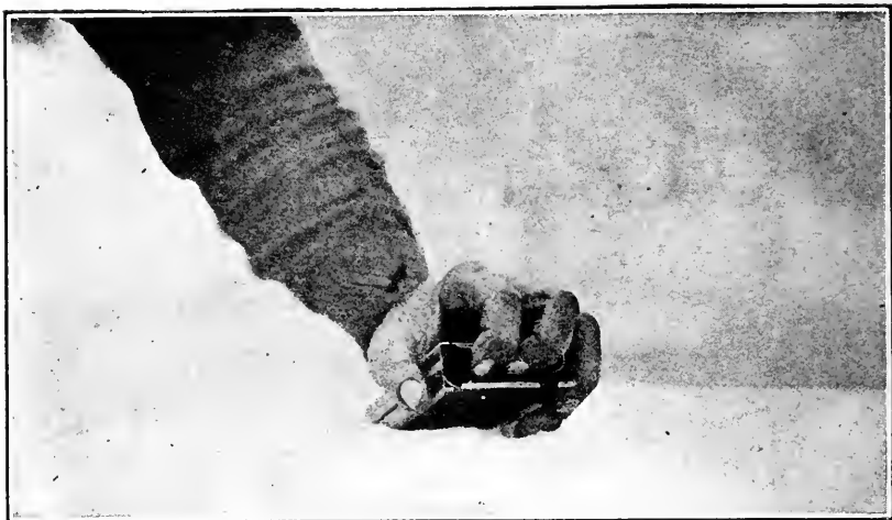
Compress magazine spring into position.
