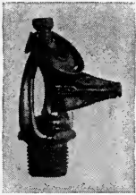
ESTY SPRINKLER WITH DEFLECTOR WORN BY VIBRA- TION.
