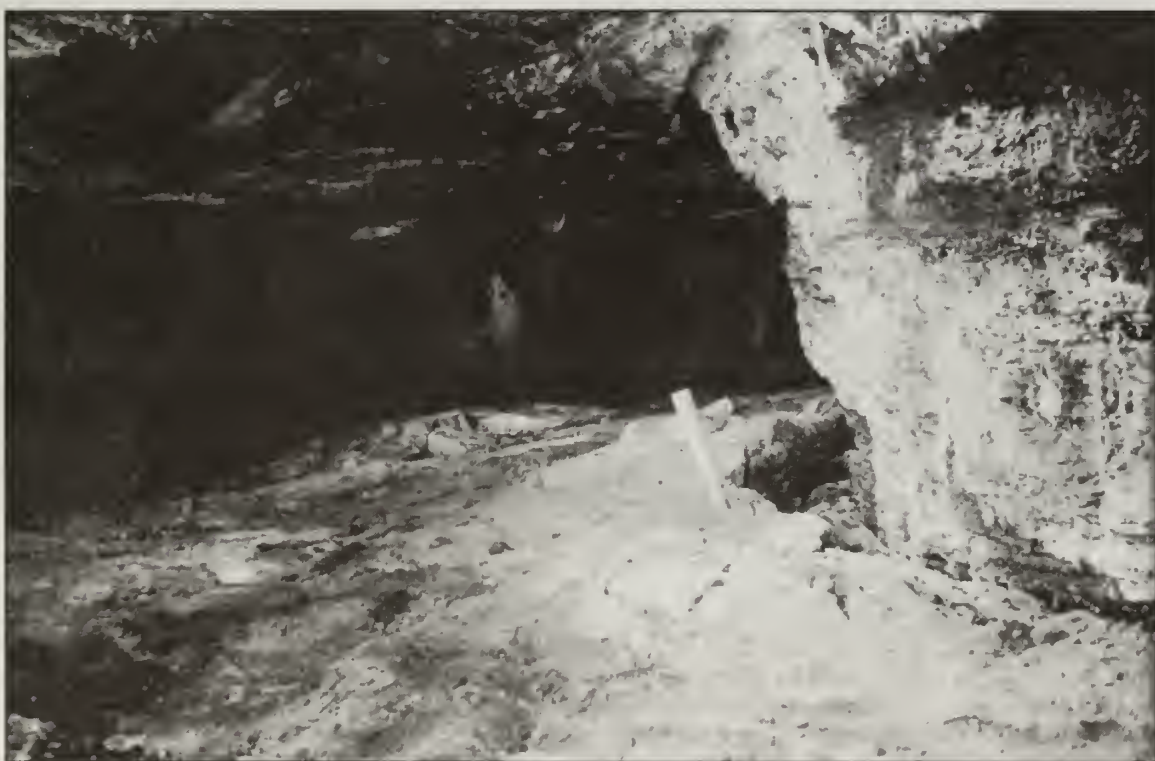
Figure 19 Floor squeeze in an underground mine in the Herrin Coal, Zeigler No. 5 Mine, Douglas County (Coal Section files, ISGS).
