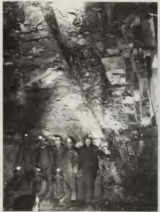
Figure 27 Highly fractured roof strata adjacent to a fault displacement, Peabody No. 44 Mine, Saline County (ISGS files).
