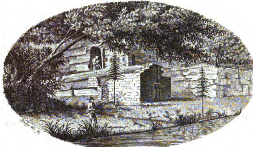
HERMITAGE at WARKWORTH.
