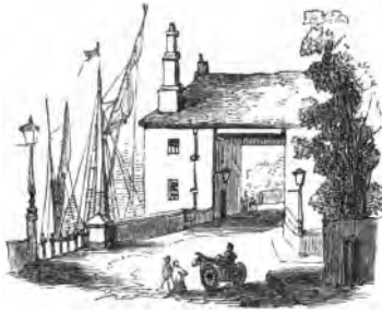
Approach to Putney Bridge.
