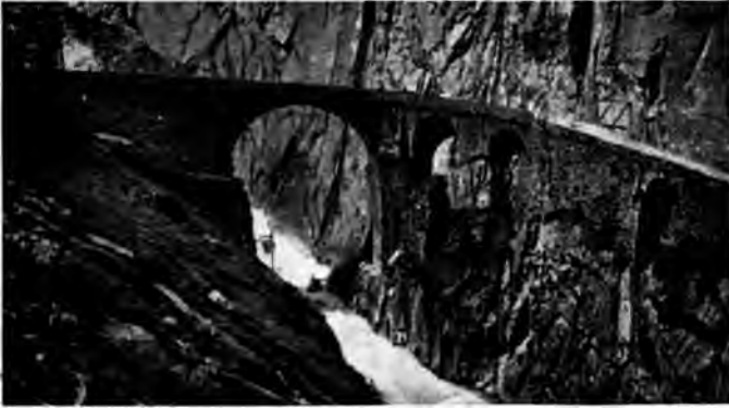
THE DEVIL'S BRIDGE
