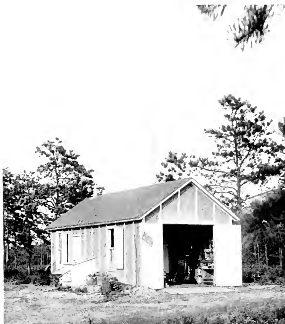
Fig. 5—Receiving test station near Riverhead, L. I. showing vertical antenna projecting through roof of building
