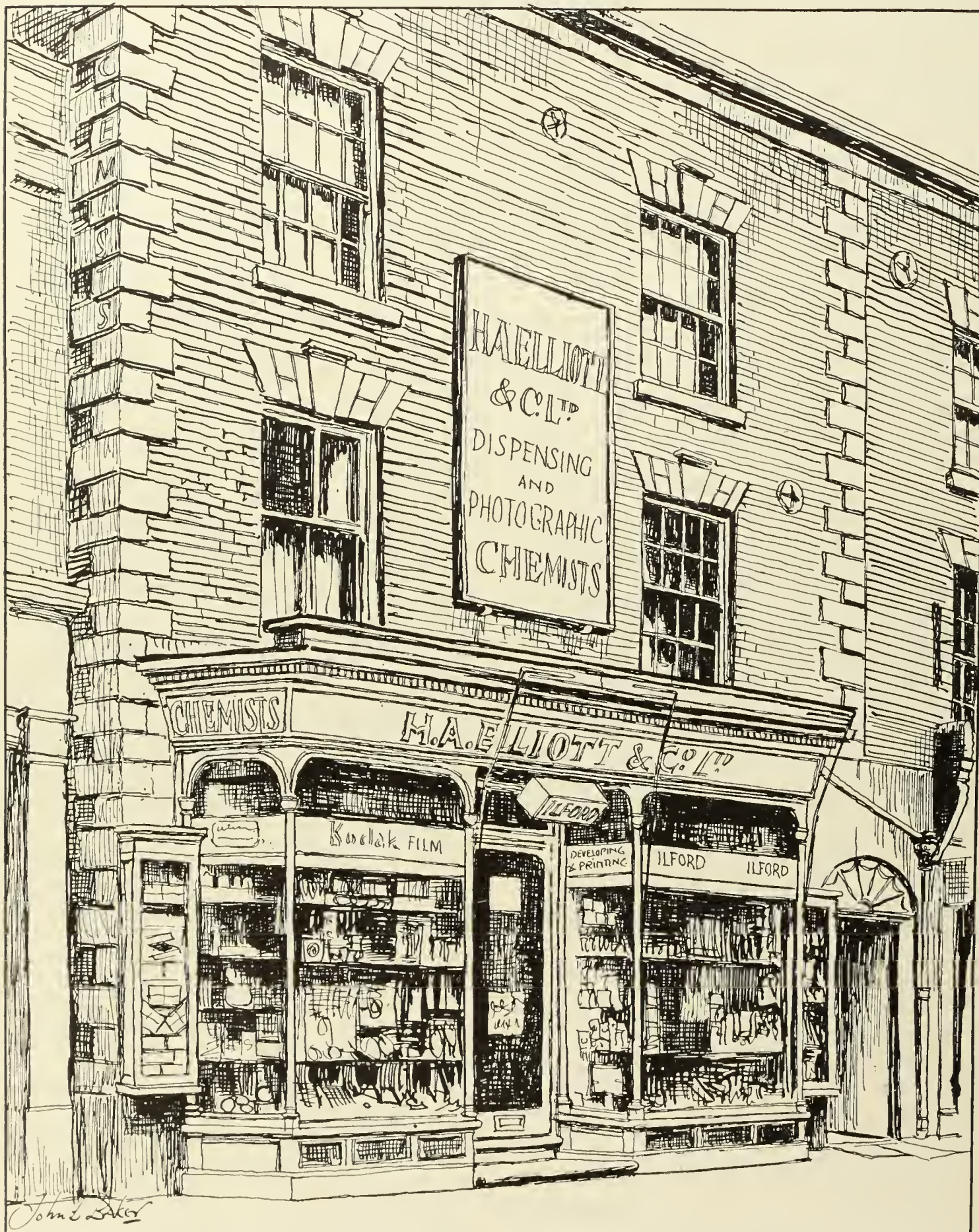
THE PHARMACY AT 59 HIGH STREET, EVESHAM
