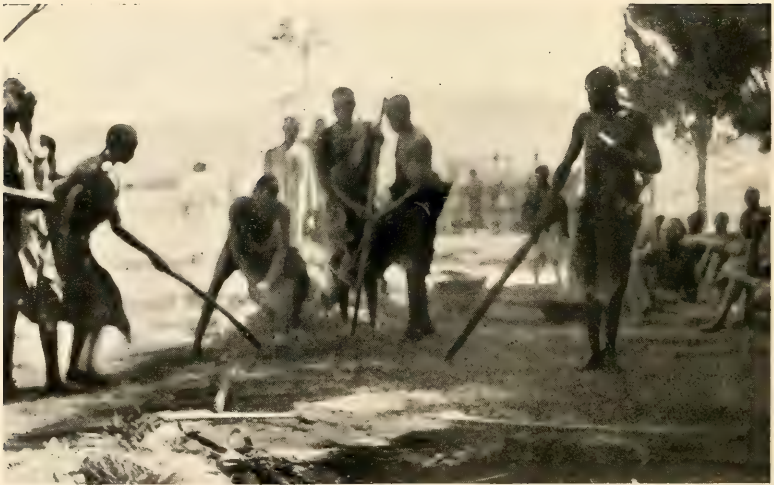
Cutting iron into small parts for smith while hot from the furnace
