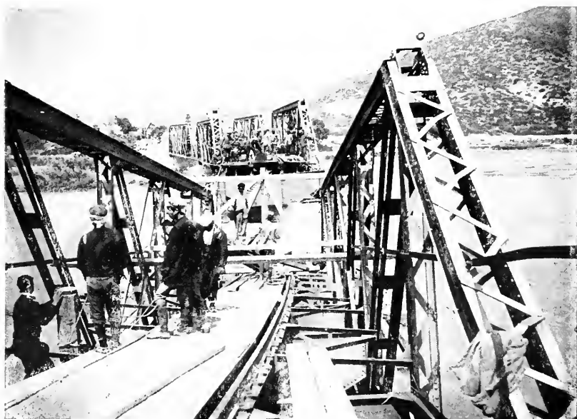
THE BRIDGE OVER THE STRUMA RIVER AT DERBEND. The centre span was blown up by the retreating Bulgarians.
