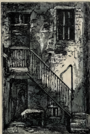
ENTRANCE TO THE OFFICES OF OLD PAUL'S WORK
