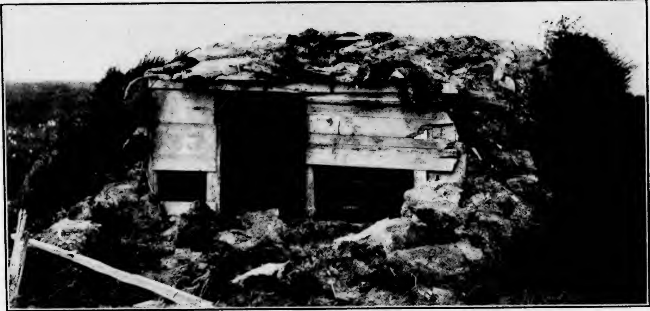
TYPE OF DWELLING OCCUPIED BY THE ESKIMOS OF THE YUKON AND KUSKOKWIM DELTA. A SKELETON FRAMEWORK OF DRIFTWOOD, COVERED WITH BLOCKS OF TUNDRA SOD. THE SOD WALLS OF THE ENTRANCE WAY HAVE FALLEN DOWN, AND MUST BE REBUILT WHEN THE HOME IS AGAIN PREPARED FOR WINTER. IN THIS 9' x 12' DWELLING LIVES A FATHER, MOTHER AND FOUR CHILDREN. WHEN THE SPRING THAWS ARRIVE THE SOD ROOF AND WALLS DRIP WATER INSIDE SO THAT THE HOME BECOMES A VERITABLE MUD-HOLE OF FILTH. THIS TYPE OF INNIE IS MUCH INFERIOR TO THOSE BUILT BY THE INNUIITS OF THE ARCTIC.
