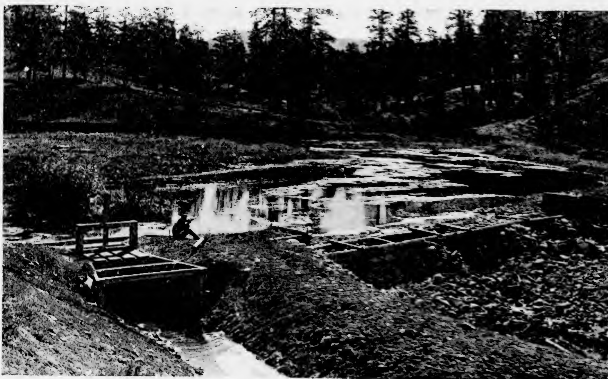
HEADWORKS OF WHEATFIELDS CREEK DITCH, BUILT BY NAVAJOS UNDER GOVERNMENT SUPERVISION.
