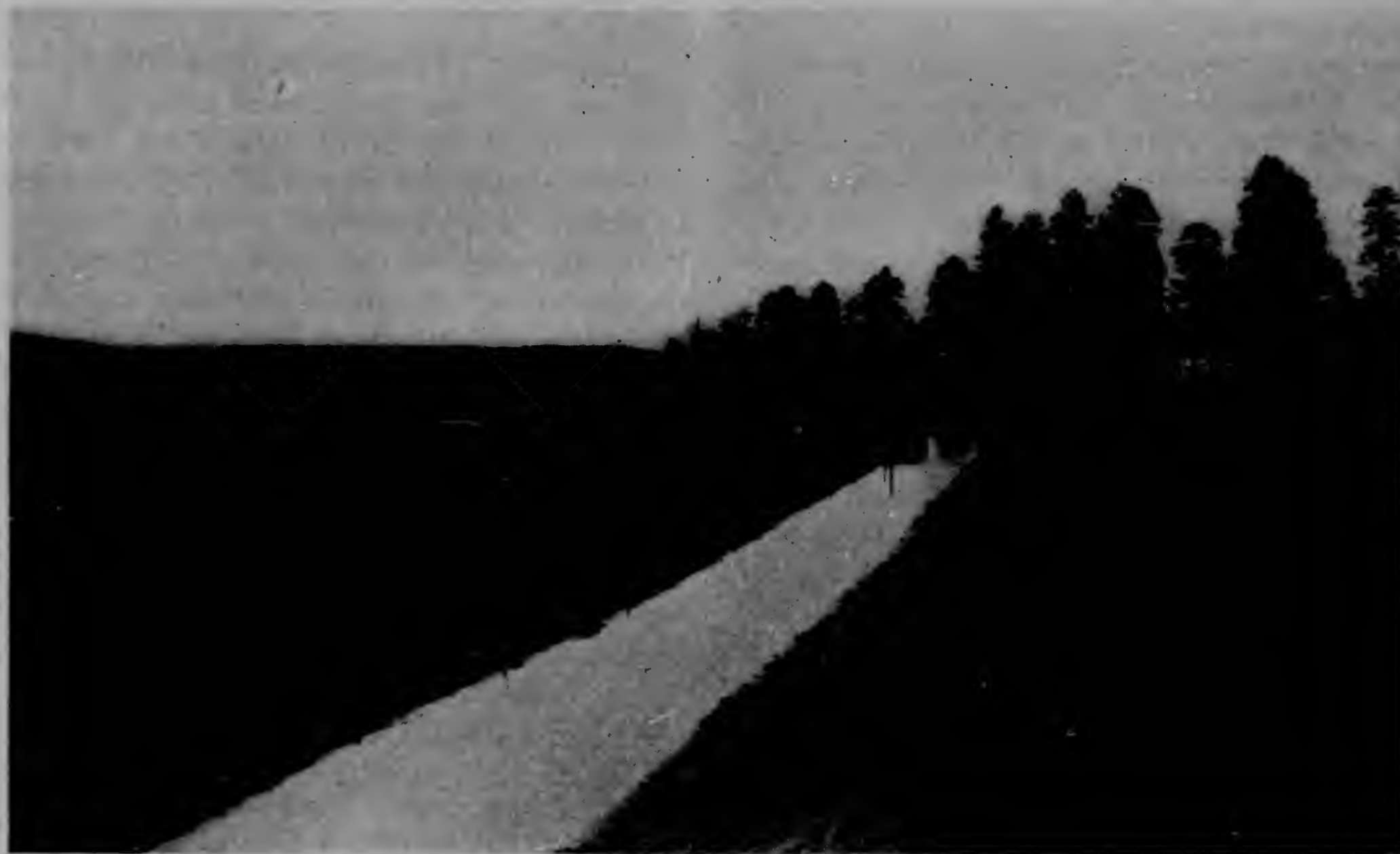
IRRIGATION FOR THE NAVAJOS, WHEATFIELDS CREEK DITCH, ARIZONA. THIS CANAL WAS BUILT BY INDIANS.
