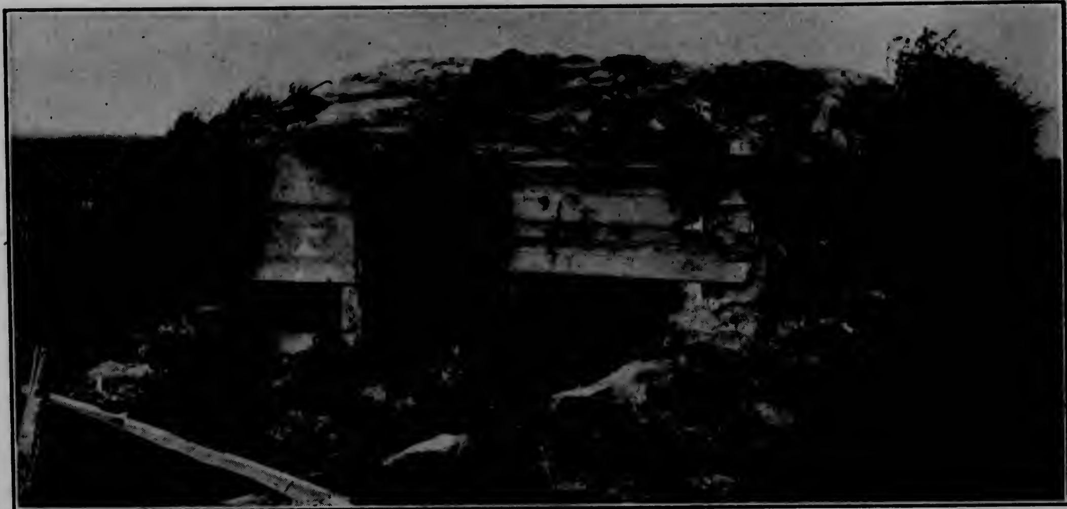
TYPE OF DWELLING OCCUPIED BY THE ESKIMOS OF THE YUKON AND KUSKOKWIM DELTA. A SKELETON FRAMEWORK OF DRIFTWOOD, COVERED WITH BLOCKS OF TUNDRA SOD. THE SOD WALLS OF THE ENTRANCE WAY HAVE FALLEN DOWN, AND MUST BE REBUILT WHEN THE HOME IS AGAIN PREPARED FOR WINTER. IN THIS 9' x 12' DWELLING LIVES A FATHER, MOTHER AND FOUR CHILDREN. WHEN THE SPRING THAWS ARRIVE THE SOD ROOF AND WALLS DRIP WATER INSIDE SO THAT THE HOME BECOMES A VERITABLE MUD-HOLE OF FILTH. THIS TYPE OF INNIE IS MUCH INFERIOR TO THOSE BUILT BY THE INNUITS OF THE ARCTIC.
