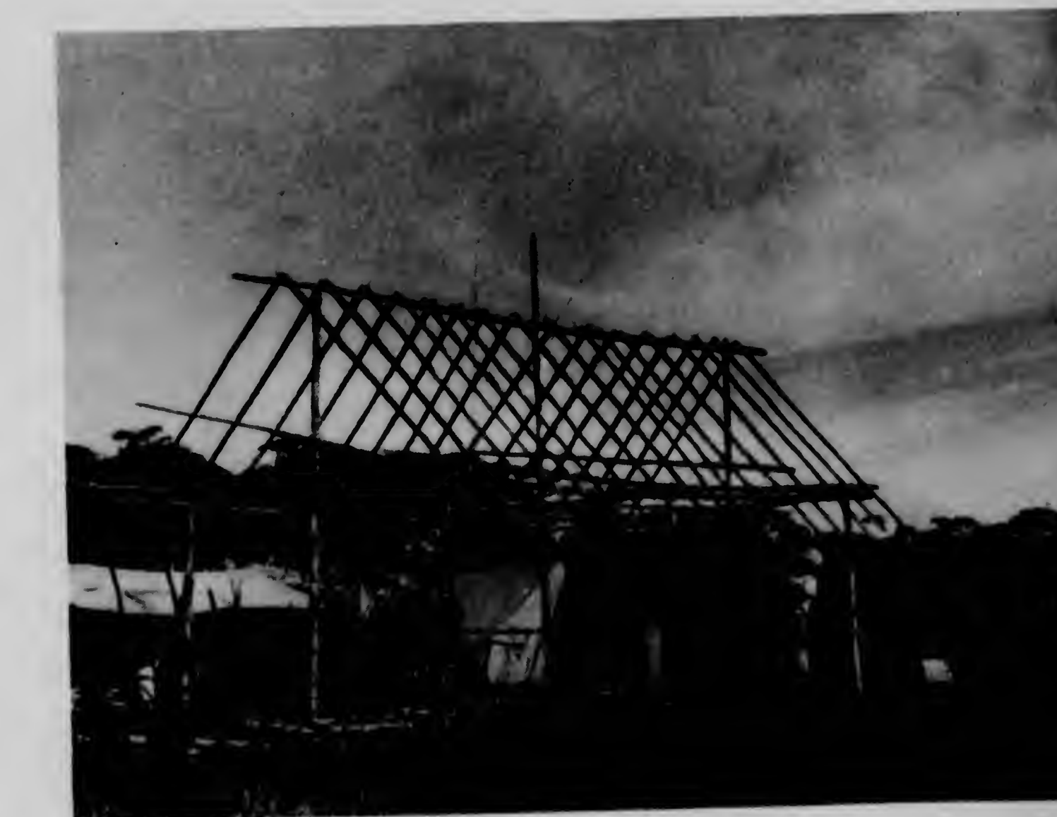
DETAILS in the kitchen's construction: posts were set deeply in the soil, holes having been gouged out with machetes; cross pieces meeting at the apex were tapered and grooved, while horizontal poles were notched, spliced and lashed securely with "bush ropes." (Below) One of the base camps in the Camarata valley showing a finished Arecuna building thatched with palm leaves
