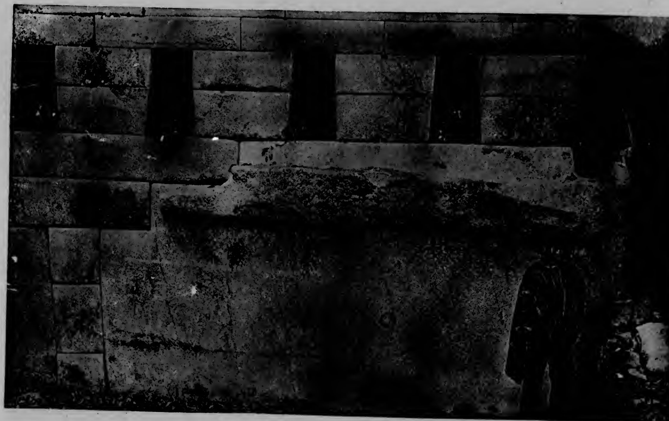
Photo by Hiram Bingham THE HEAVIEST STONE BLOCK IN A MACHU PICCHU WALL The interior face of the same stone and the ornamental niches in the east wall of the Chief Temple. The hole in the upper right-hand corner was undoubtedly for the admission of the beam which supported the roof of this temple.
