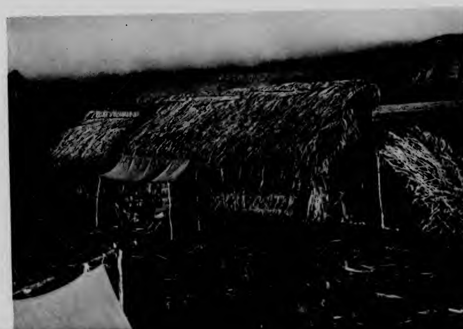
DETAILS in the kitchen's construction: posts were set deeply in the soil, holes having been gouged out with machetes; cross pieces meeting at the apex were tapered and grooved, while horizontal poles were notched, spliced and lashed securely with "bush ropes." (Below) One of the base camps in the Camarata valley showing a finished Arecuna building thatched with palm leaves
