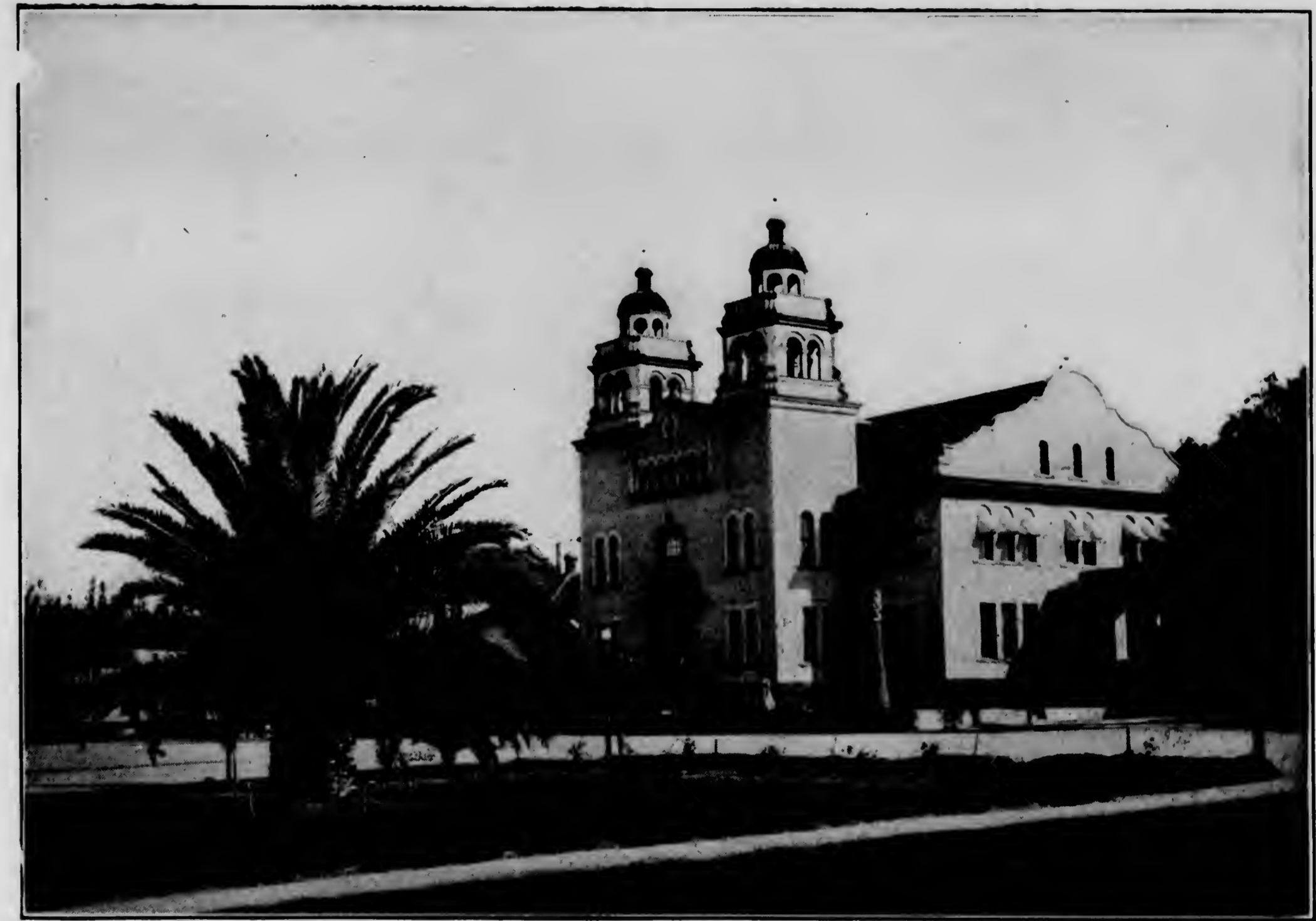
Main School Building
