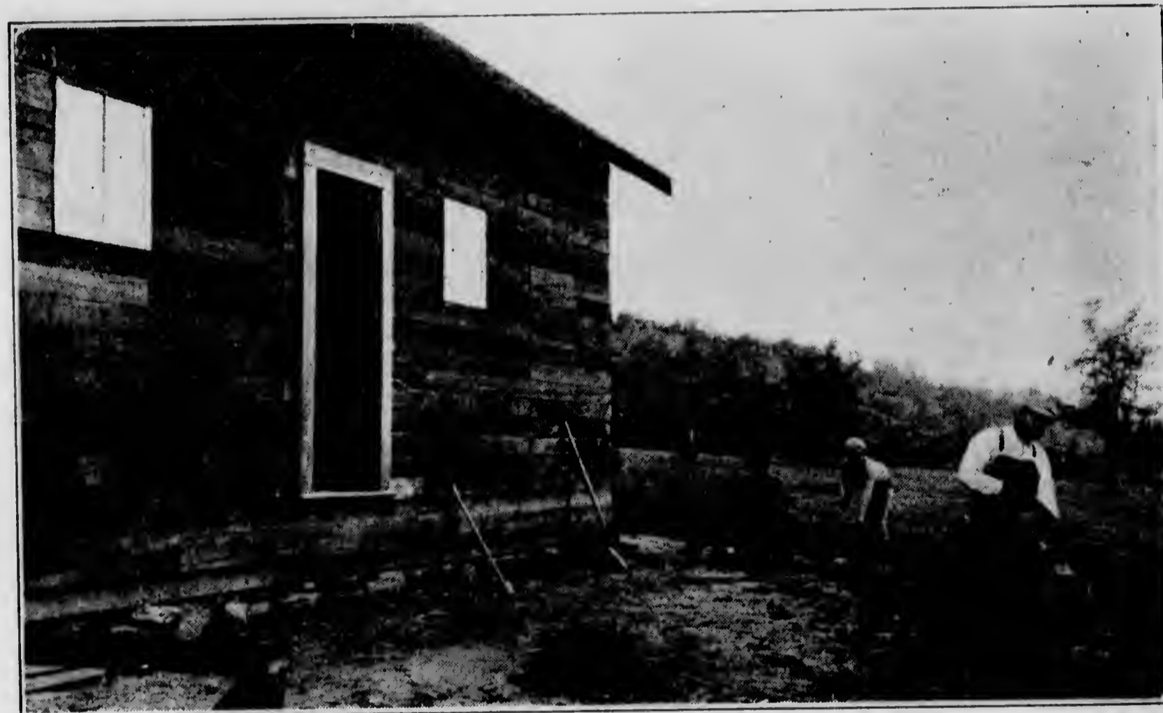
Building a porch for the boys' dormitory.
