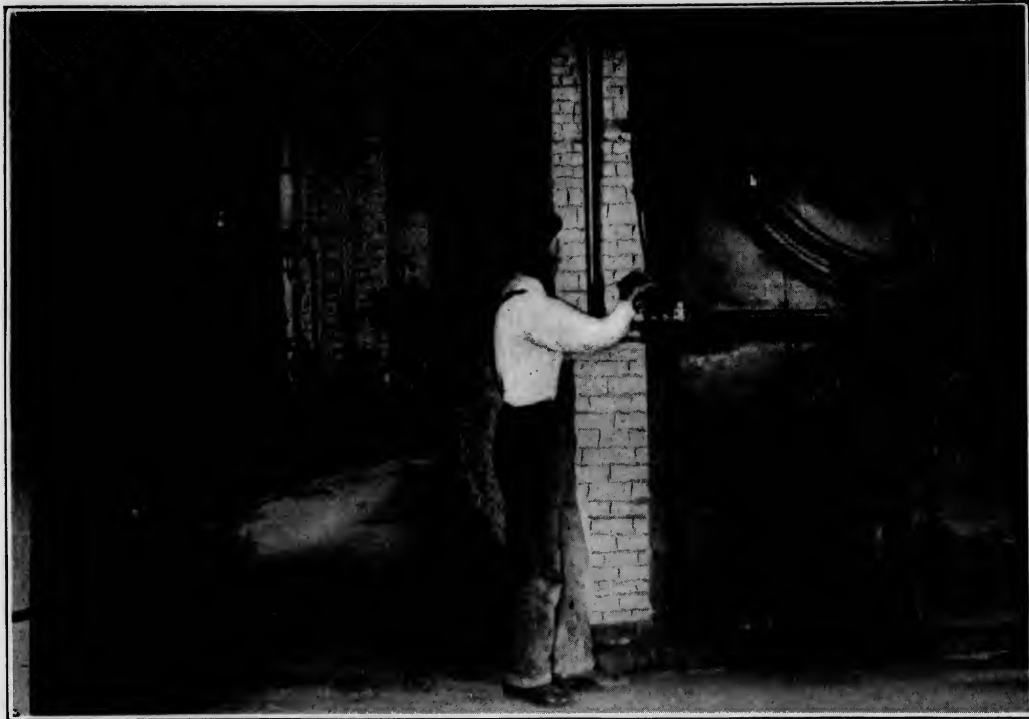
In the Boiler House
