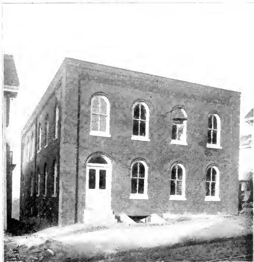
THE SUB-STATION ON PARK STREET
