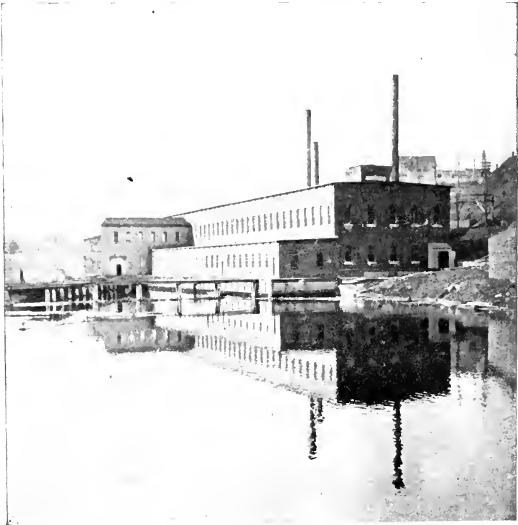
POWER STATION ON THE PENOBSCOT AT VEAZIE
