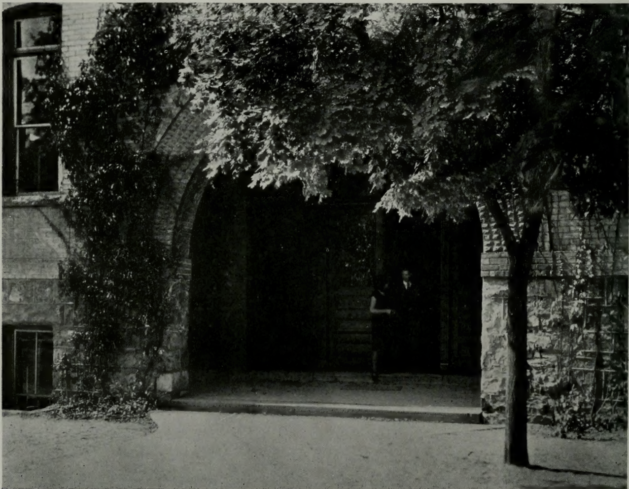
EAST ENTRANCE TO COLLEGE BUILDING
