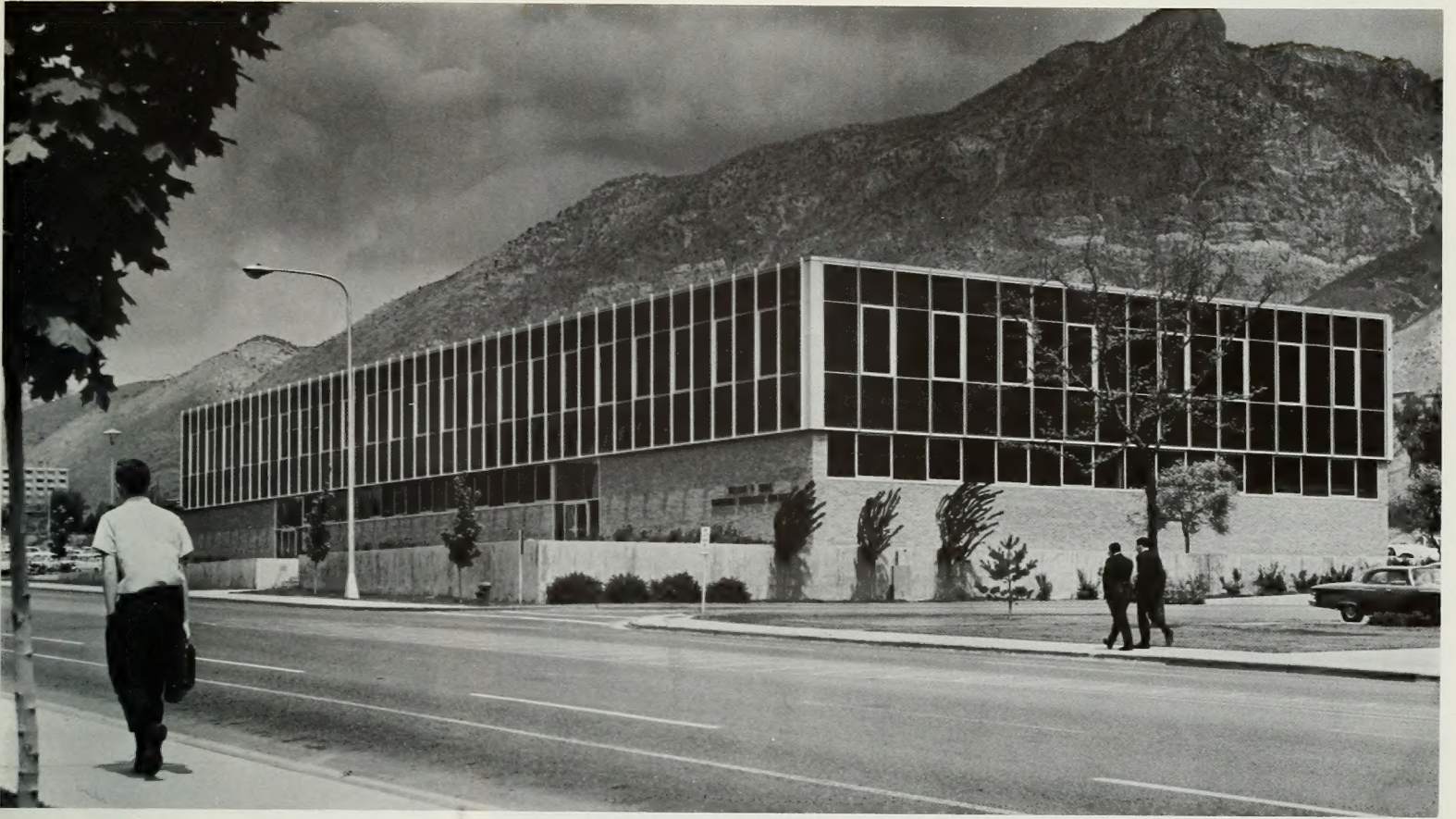
The William H. Snell Industrial Education Building offered facilities used by a large part of the students enrolled in the college.
