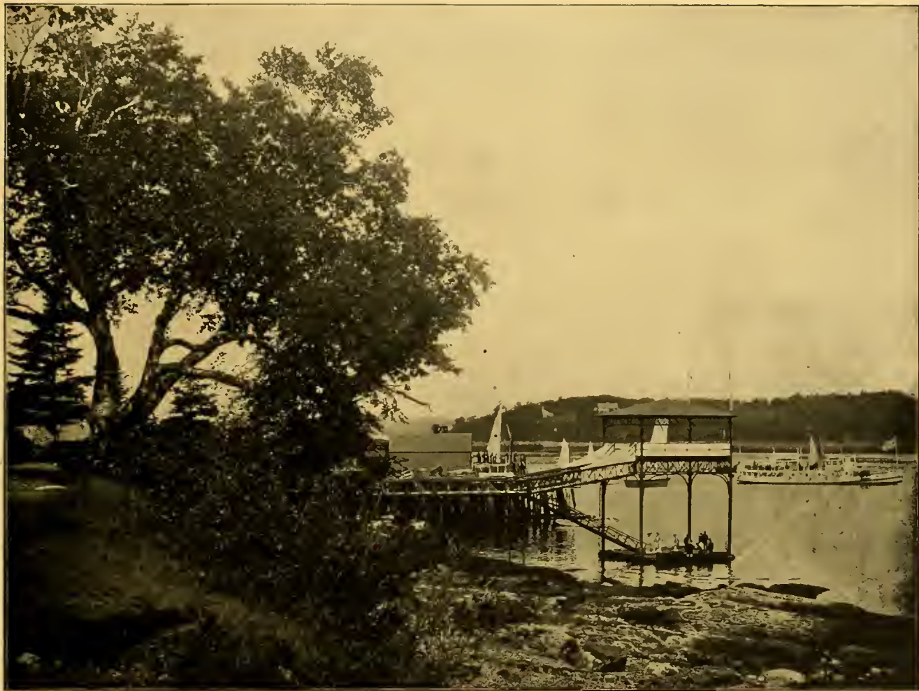
STEEL PIER OF THE MOUNT DESERT READING ROOM AND HARBOUR VIEW
