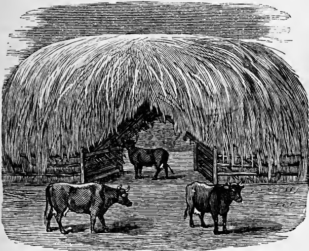
Fig. 59—THE ARCHWAY UNDER THE STACK COMPLETE.
