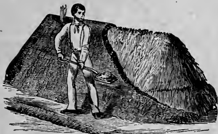
Fig. 243.—COVERING HEAP WITH EARTH.
