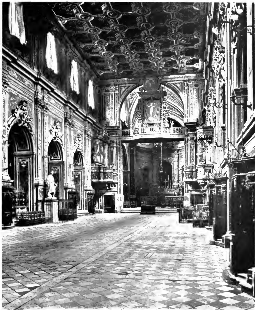
Fig. 41.—Naples. Church of the Carmine. Interior.
