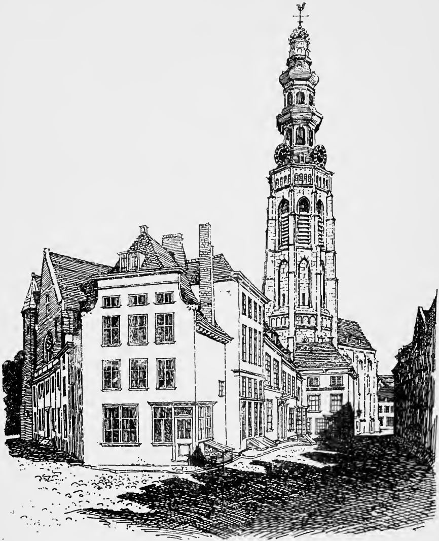
Fig. 101.—Middelburg. The Abbey Steeple. (“Lang Jan.”)
