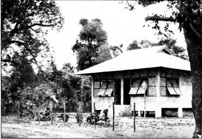
Bureau of Education, Manila, P. I. A permanent barrio school building.
