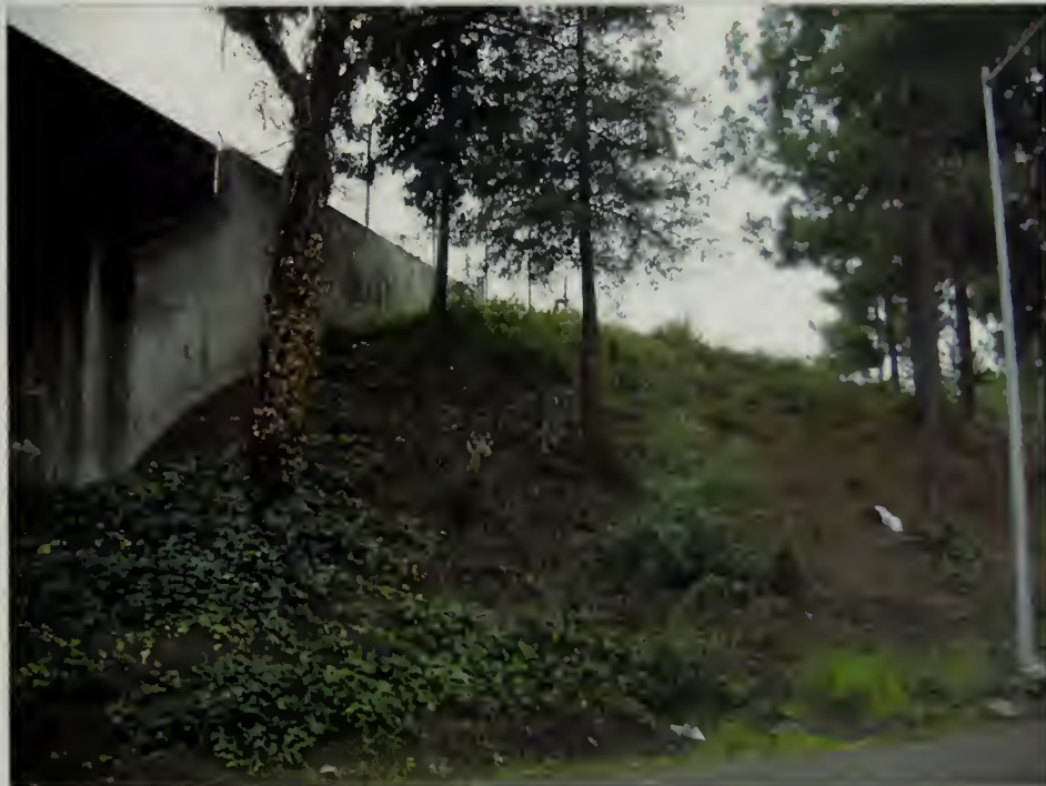
Chabot Road Overpass
