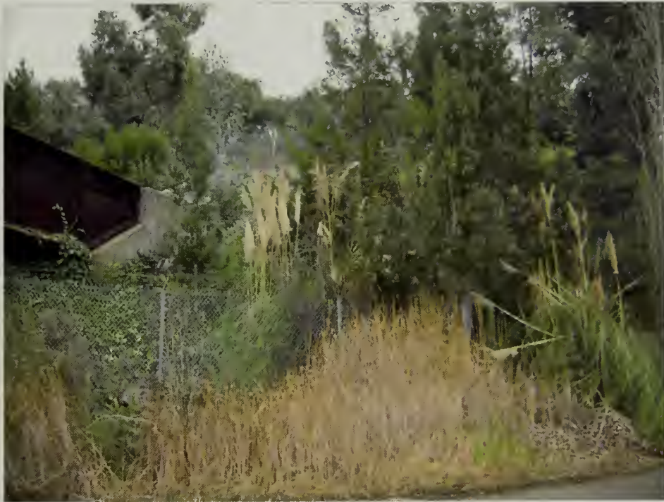
Chabot Road Overpass
