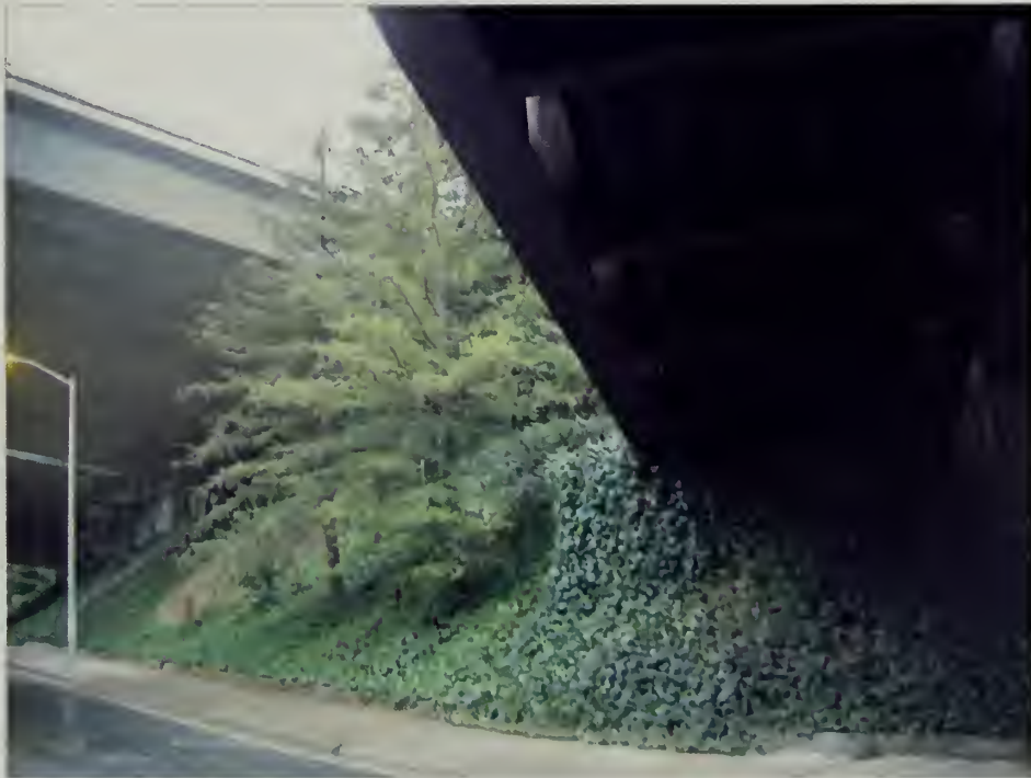
Golden Gate Avenue Overpass
