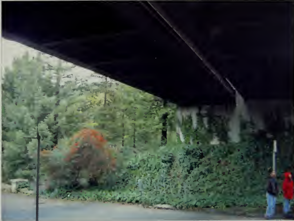
Golden Gate Avenue Overpass
