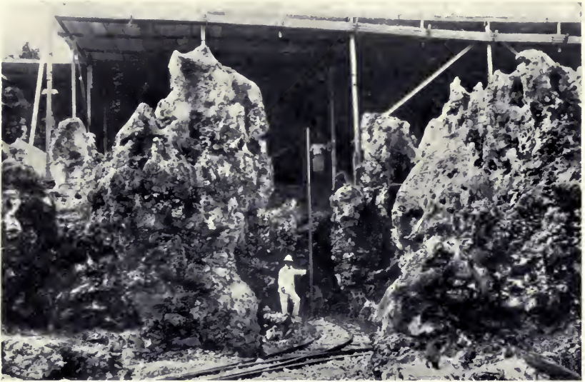
Ocean Island Phosphate Workings. Coral pinnacles after most of the phosphate has been removed. A few feet more phosphate available below rail level.
