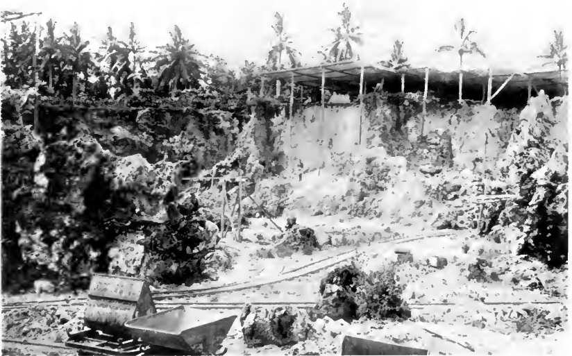
Ocean Island Phosphate Workings. Foreground: Most of the phosphate has been removed exposing the coral limestone pinnacles. Background: Phosphate deposit is intact and exists mostly in the form of gravel with occasional large boulders of phosphate.
