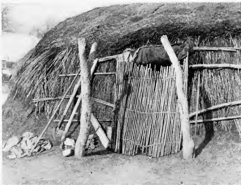
Fig. 3. Oldest Type of House showing a Door constructed with Rows of Wrapped Weaving.
