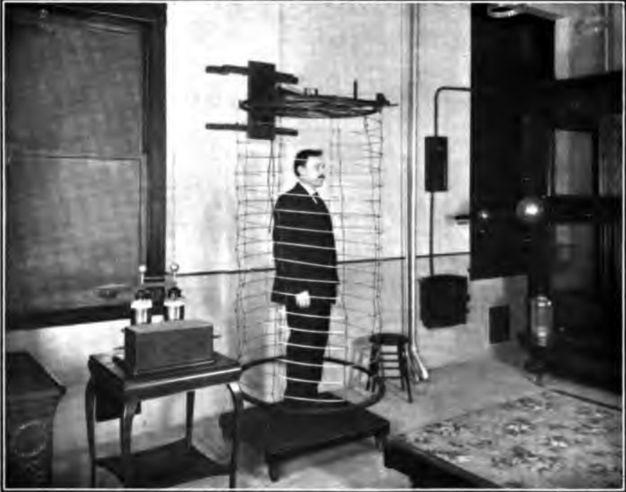
STATIC ELECTRICAL DEPARTMENT.
