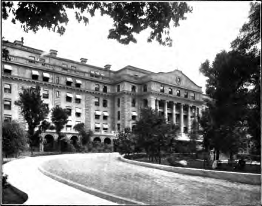
NEW MAIN BUILDING.
