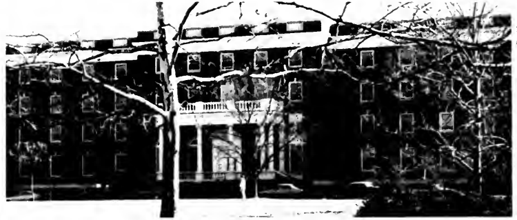
Thomas Jefferson Hall residence
