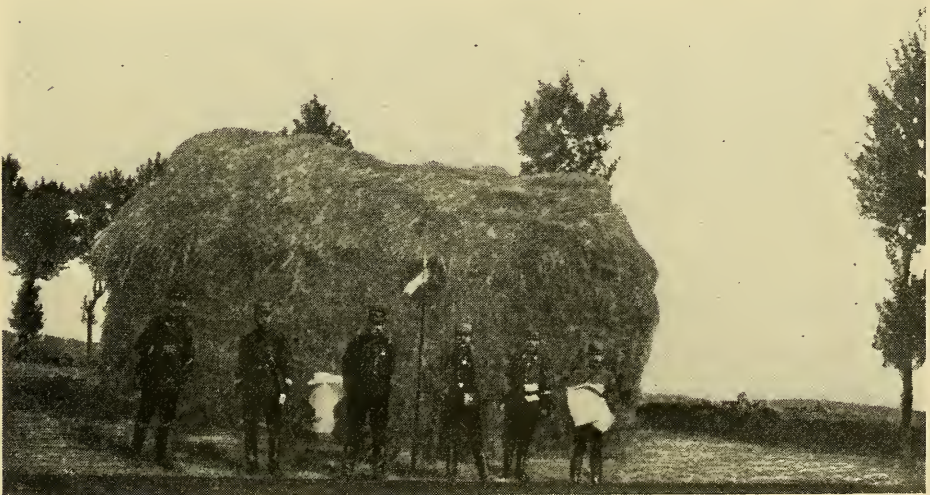
General de Dartein's Temporary Headquarters at Marcilly
