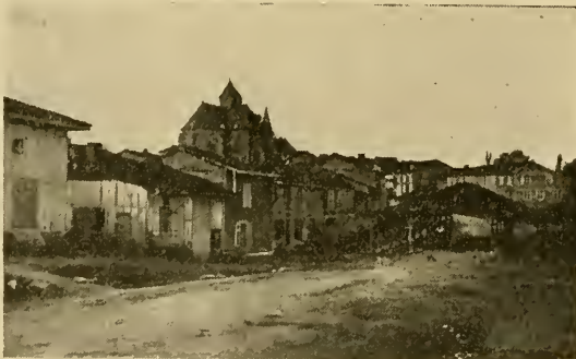
View of Cheminon (Looking West)
