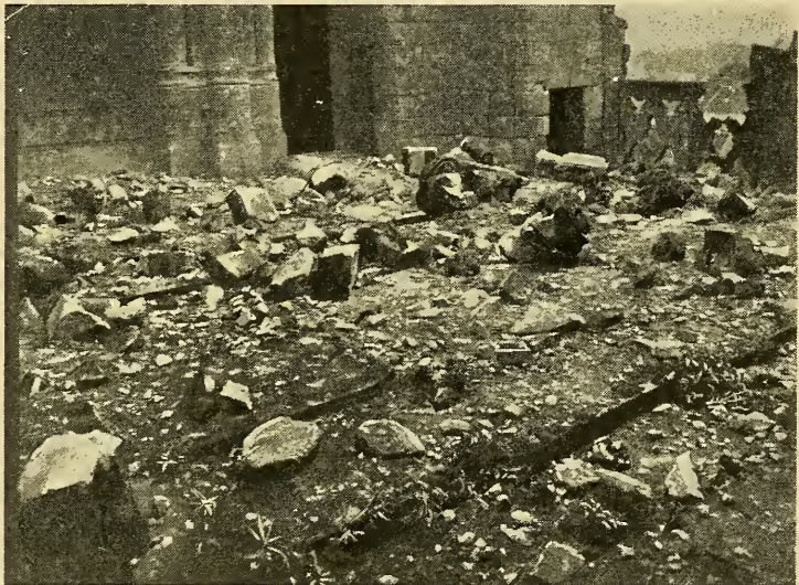
Debris at the Foot of the Cathedral Towers. (Photo by M. H.)
