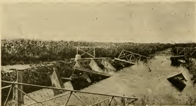
Destroyed Bridge over the Morin
