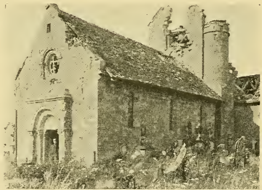
Exterior of the Church
