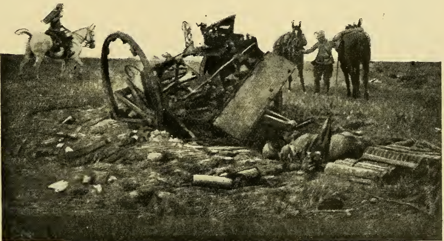
German Field-piece destroyed near Poligny
