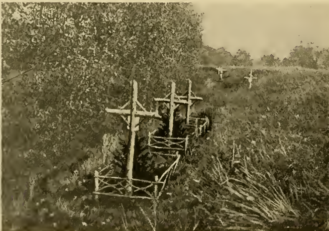
Trenches and Graves near the Level-Crossing at Normée
