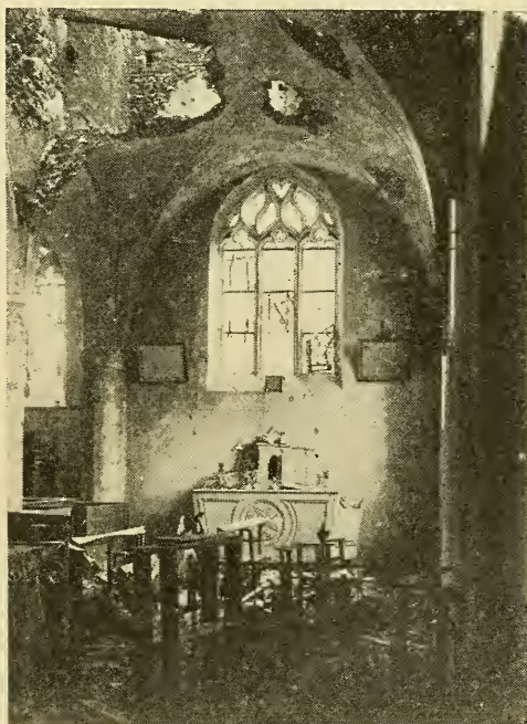
Interior of Montceaux Church
