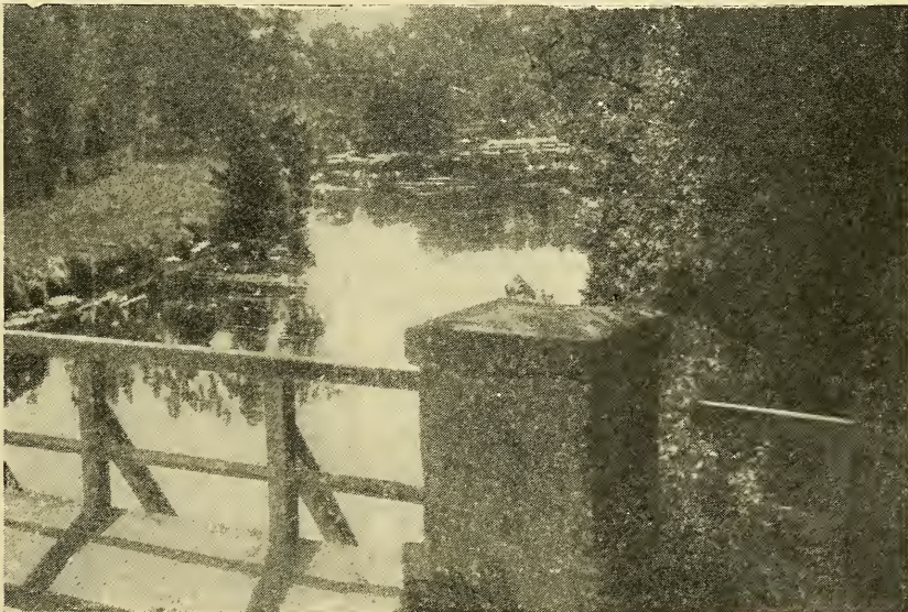
Bridge over the Morin
