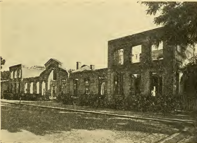
Interior of the Burned Station (September, 1914)
