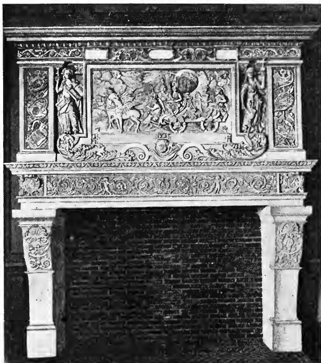
Chimney Piece in the Prefecture (XV th Century)
