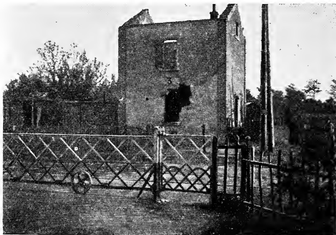
Level-Crossing at Normée
