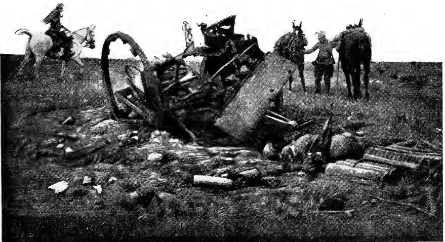
German Field-piece destroyed near Poligny
