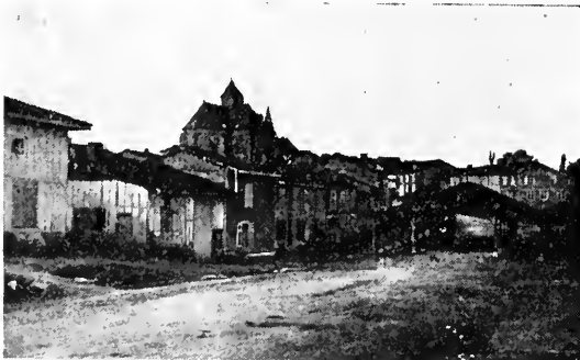
View of Cheminon (Looking West)
