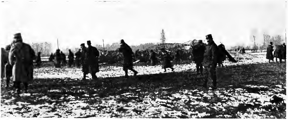
Debris of the Zeppelin Brought Down at Revigny
