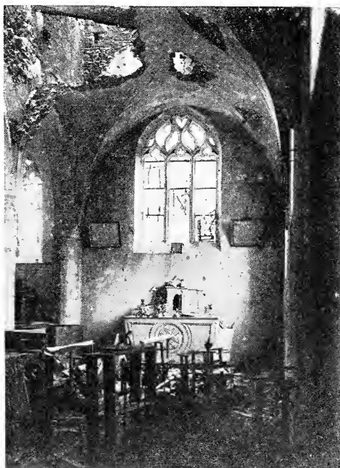
Interior of Montceaux Church
