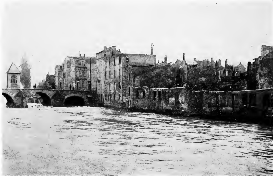
Environs of Nôtre-Dame Bridge after an Air Raid
