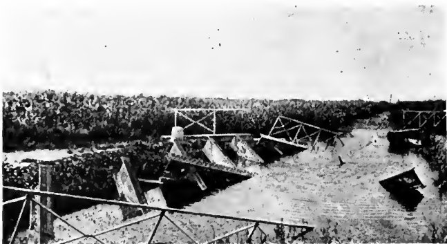
Destroyed Bridge over the Morin
