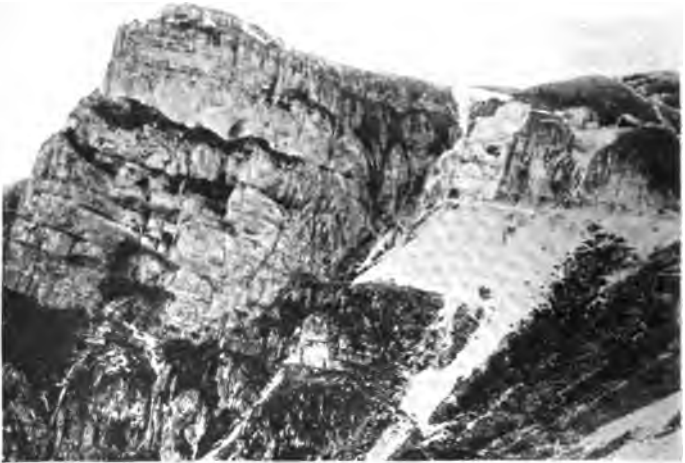
FIG. 123—New Italian military road zigzagging up a steep precipice on the slope of Monte Baldo. Several tunnels may be noted within the space of a few hundred yards.
