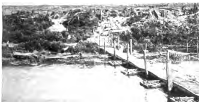
FIG. 10—A canal used as a defense line and crossed by a temporary footbridge. (Belgian official photograph.)
