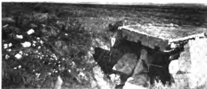
FIG. 54—Partially destroyed concrete machine-gun shelter in a trench of the Hindenburg Line southeast of Arras. From this shelter a deadly grazing fire swept the exposed surface of the barren Somme plain.
