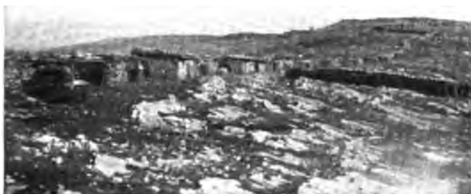
FIG. 147—Defensive position on western margin of the Carso north of Monfalcone. The barren aspect of the limestone country is apparent, and stone breastworks and shelters replace trenches and underground dugouts. (Italian official photograph.)
