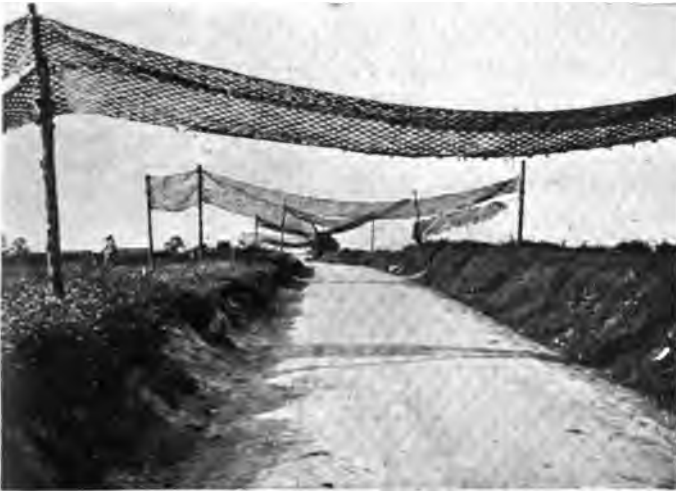
FIG. 31—German camouflage of a road across the Somme battlefield. Roads on the white chalk of the barren plain are readily visible for great distances; hence the necessity for concealing them by strips of this type, which prevent effective observation from enemy captive balloons or other points near the horizon. (French official photograph.)
