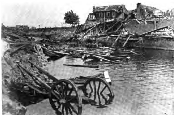
FIG. 44—The Oise Canal at Chauny, part of the Oise valley barrier. Note that the bridge has been destroyed and that material has been lost in attempting the passage. (French official photograph.)
