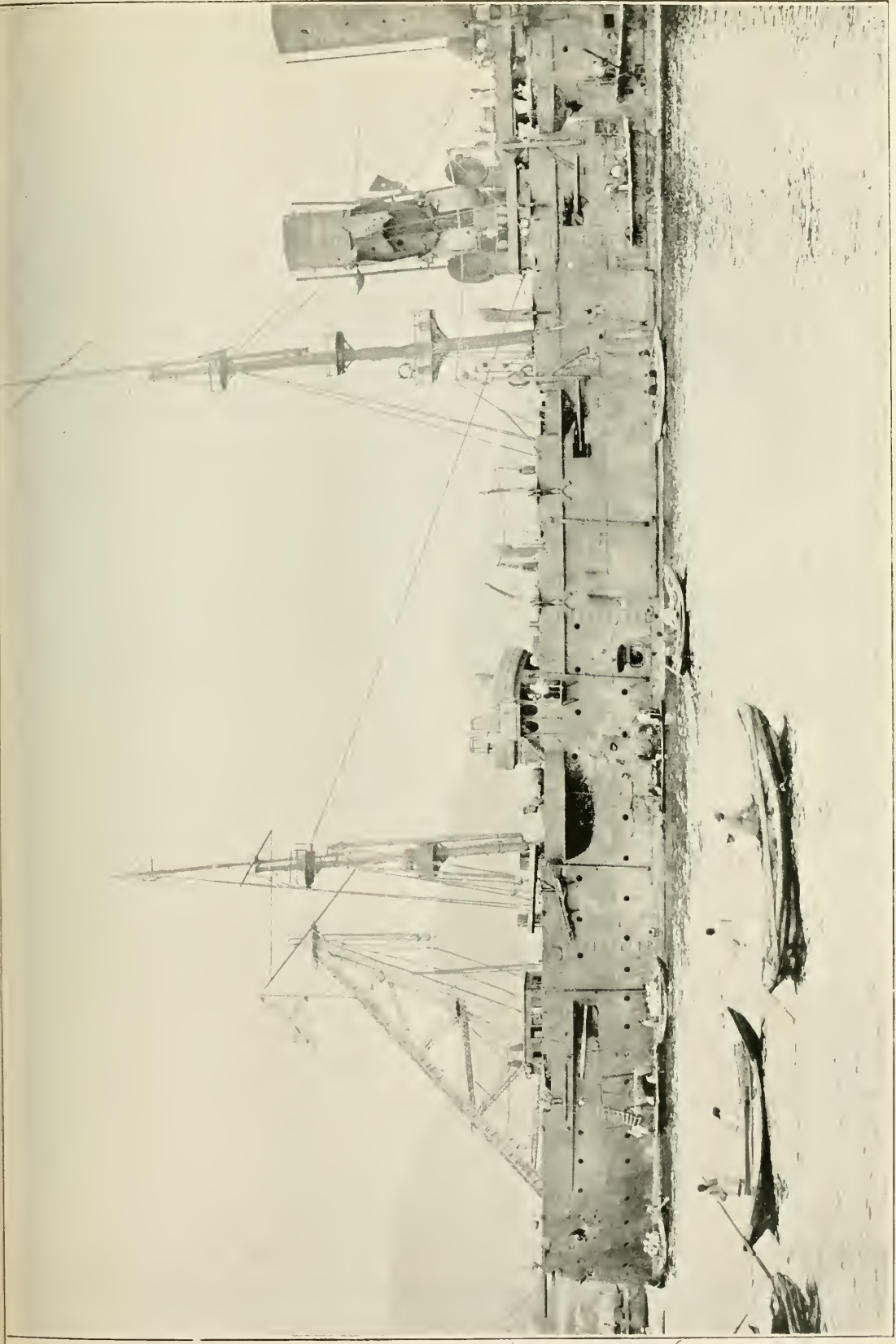
AFTER-PART OF THE CRUISER "ROSSIA." GENERAL VIEW OF DAMAGE RECEIVED.
