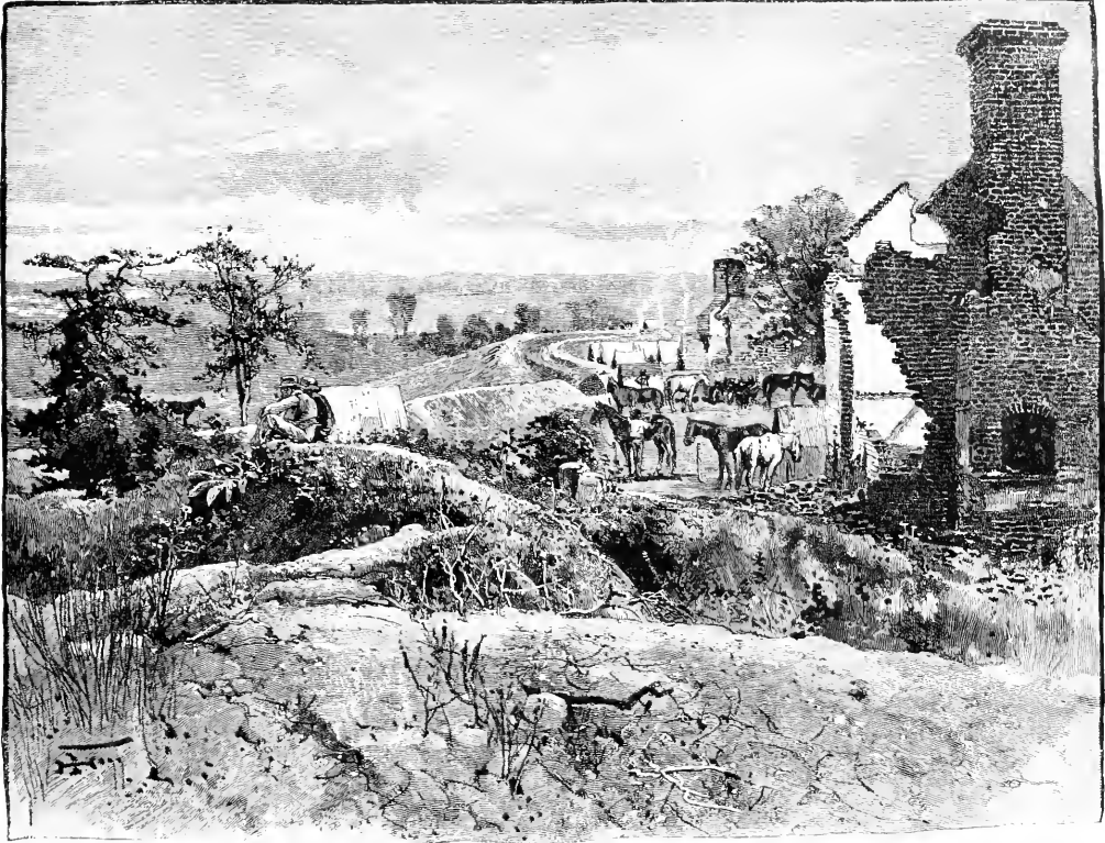
CONFEDERATE WORKS ON WILLIS'S HILL, NOW THE SITE OF THE NATIONAL CEMETERY. FROM A WAR-TIME PHOTOGRAPH.
