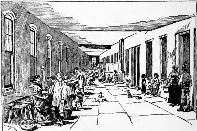
Flagged Hallway in the "Big Flat."
