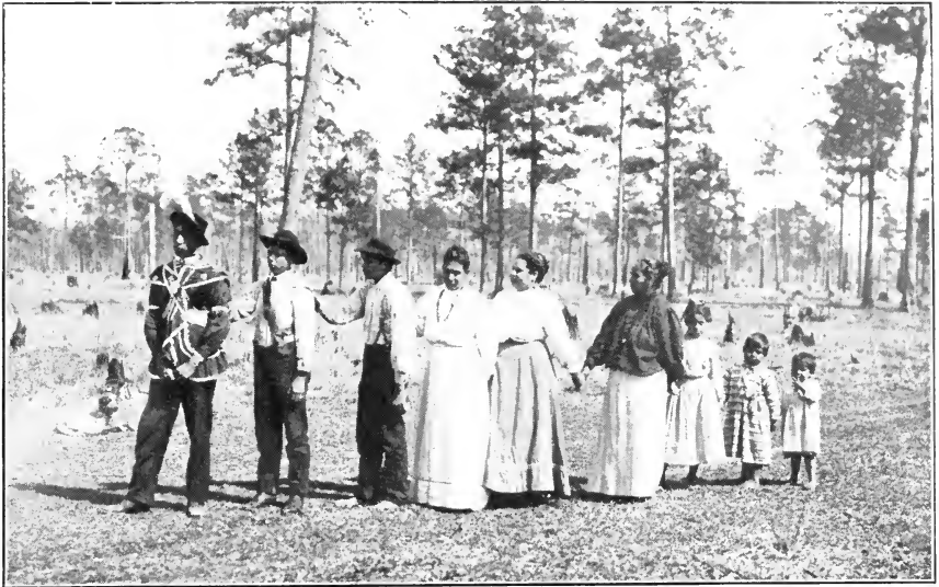
READY TO BEGIN
