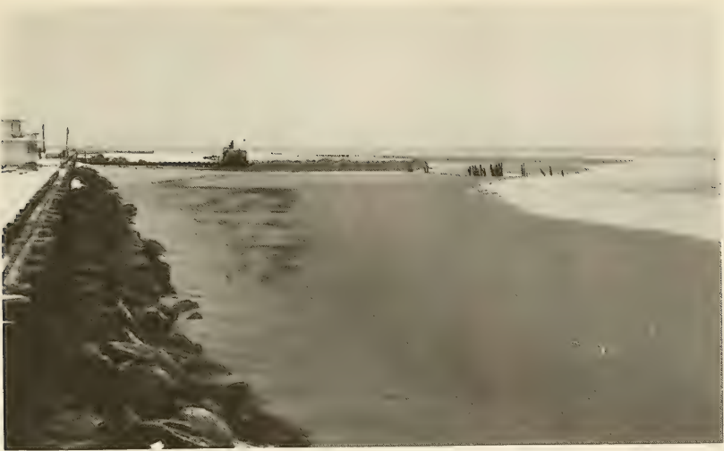
Figure 9. Strathmere bulkhead, view toward profile line 3, February 1974.
