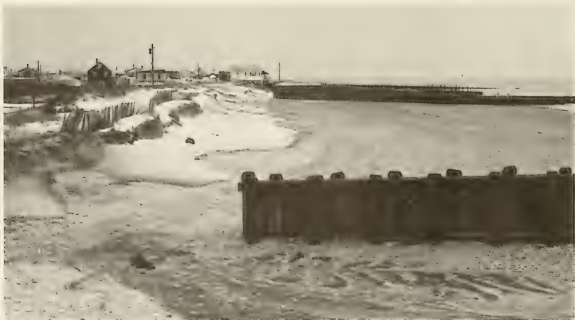
Figure 8. Flanked groin at south end of Strathmere, February 1974.
