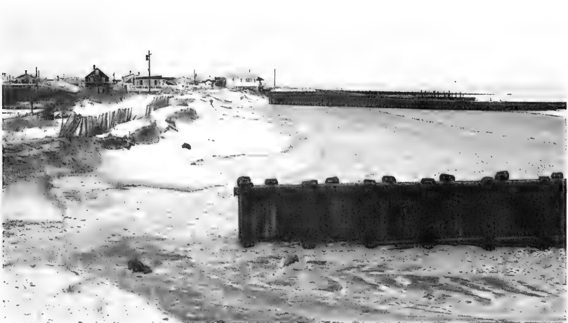
Figure 8. Flanked groin at south end of Strathmere, February 1974.
