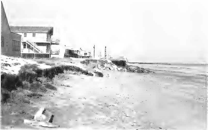
Figure 12. Eroded beach south of bulkhead in Sea Isle City, February 1974.
