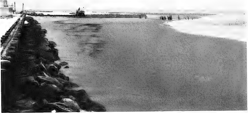
Figure 9. Strathmere bulkhead, view toward profile line 3, February 1974.
