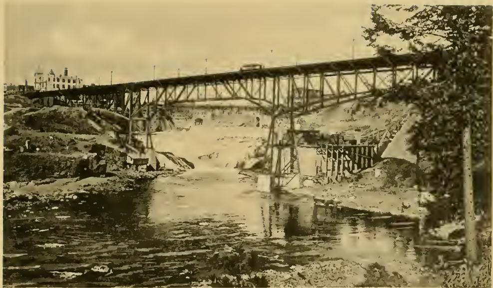
MONROE STREET BRIDGE.
