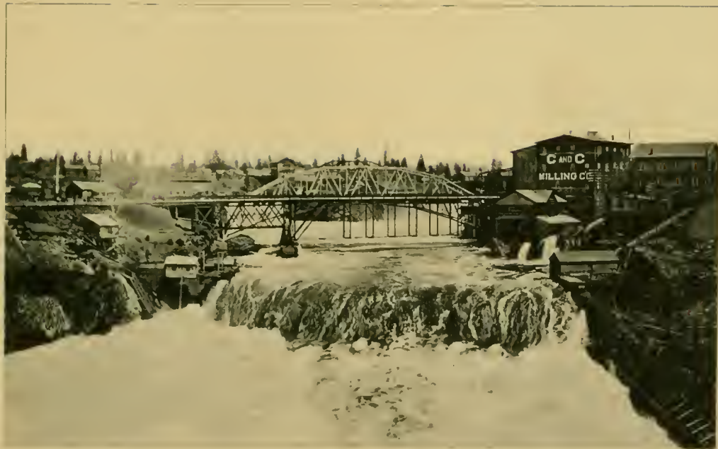
VIEW OF THE LOWER FALLS AND POST STREET BRIDGE.
