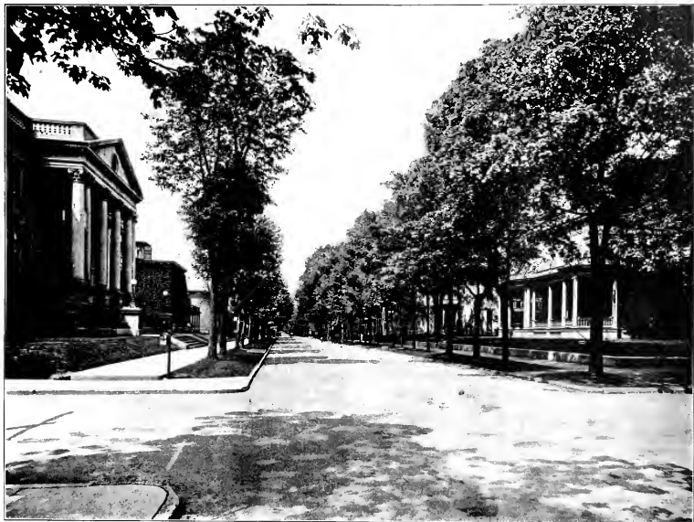
WEST WAYNE STREET, FROM WEBSTER STREET
