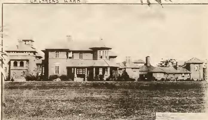
SIDE VIEW OF EXTERIOR
