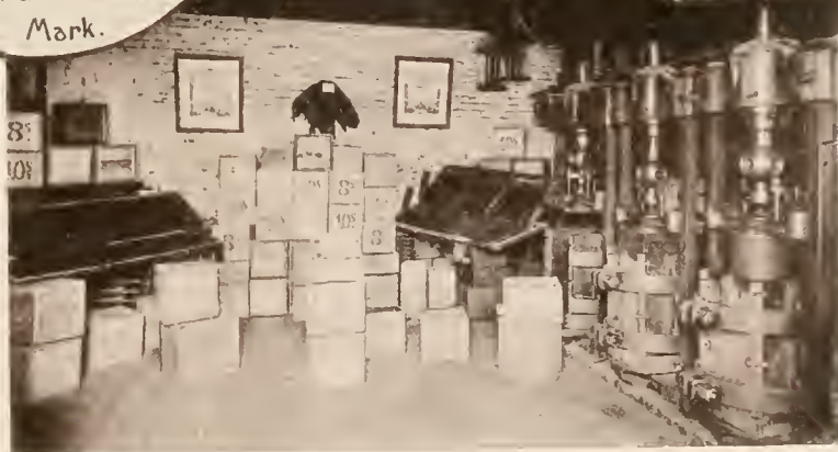
Interior of Factory.
