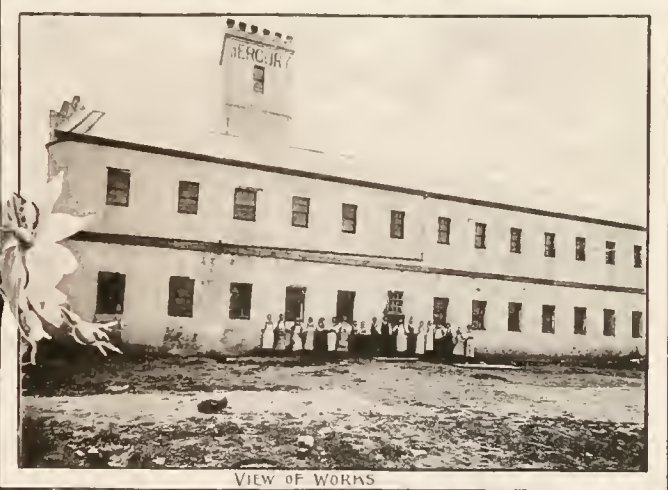
VIEW OF WORKS
