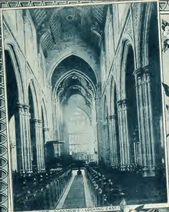
• NAVE ST ANDREW'S • LOOKING EAST •
