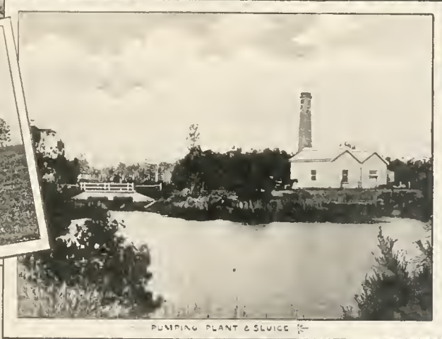
PUMPING PLANT & SLUICE
