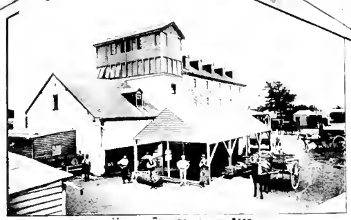
VIEW OF BREWERY, LOOKING EAST.
