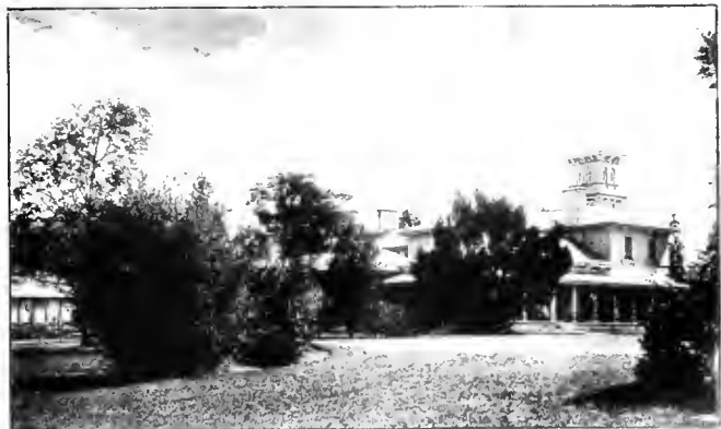
A VIEW OF THE RESIDENCE
