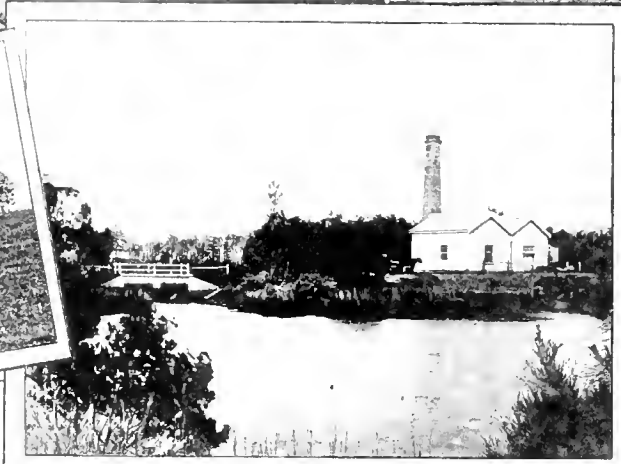
PUMPING PLANT & SLUICE
