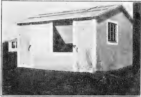
Curtain-Front Laying Competition House, Connecticut Agricultural College, Storrs. All These Houses Are New, and All Alike
