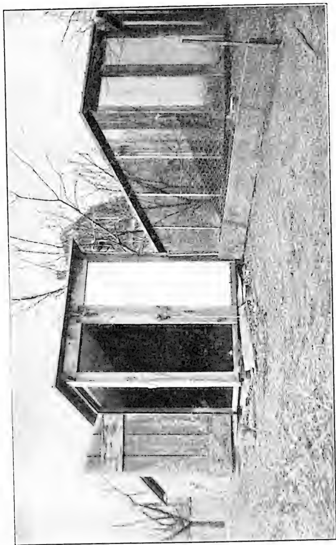
Simple but Efficient Duck Houses. Cloth Front Curtains Swinging Upward and Inward
