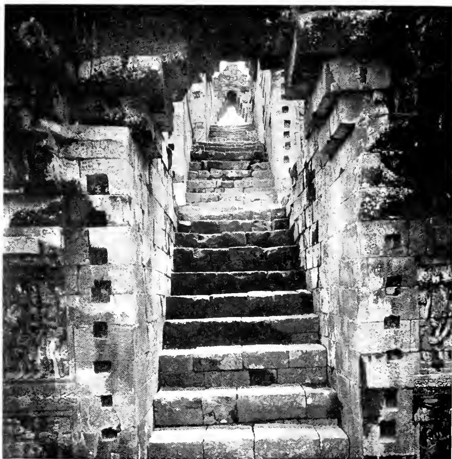
2 STAIRCASE AT BORO BUDUR (NORTH SIDE)
