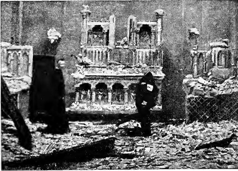
Interior of a Church at Termonde.
