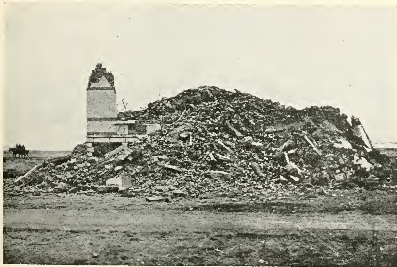
40. A GERMAN VILLA, PREPARED FOR HEAVY HOWITZERS, DESTROYED BY THE BELGIAN ENGINEERS. ( Page 152 )
