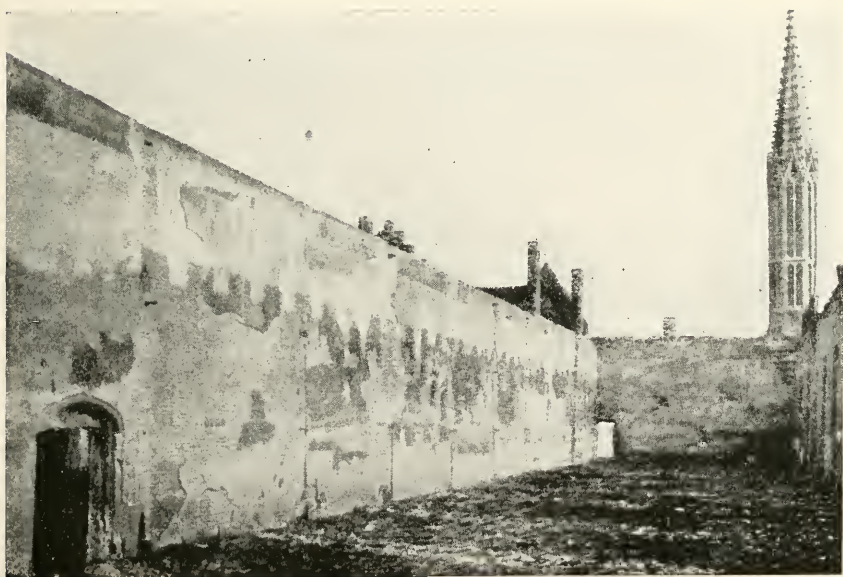
43. THE SAME CHAMBER IN NOVEMBER, 1915.
