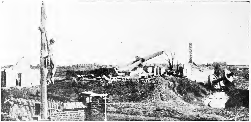
53. FARMHOUSES AND COTTAGES AND WINDMILLS DEMOLISHED. ( Page 235 )
