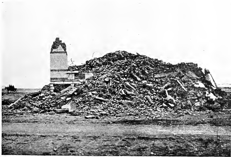
40. A GERMAN VILLA, PREPARED FOR HEAVY HOWITZERS, DESTROYED BY THE BELGIAN ENGINEERS. ( Page 152 )
