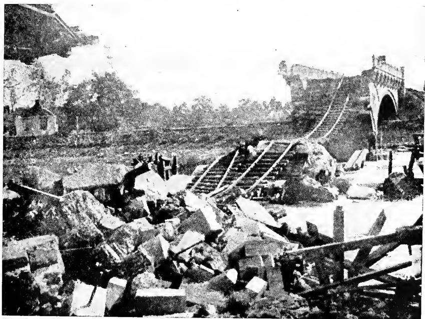
26. THE DUFFEL BRIDGE OVER THE NÈTHE, DESTROYED BY THE BELGIANS. (Page 114)
