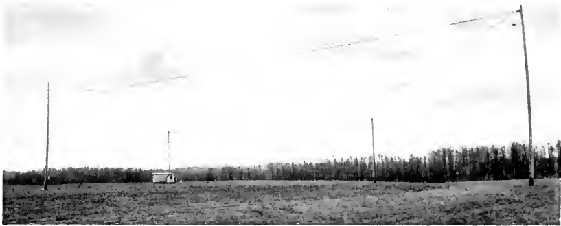
Fig. 22—An experimental horizontal diamond-shaped antenna.
