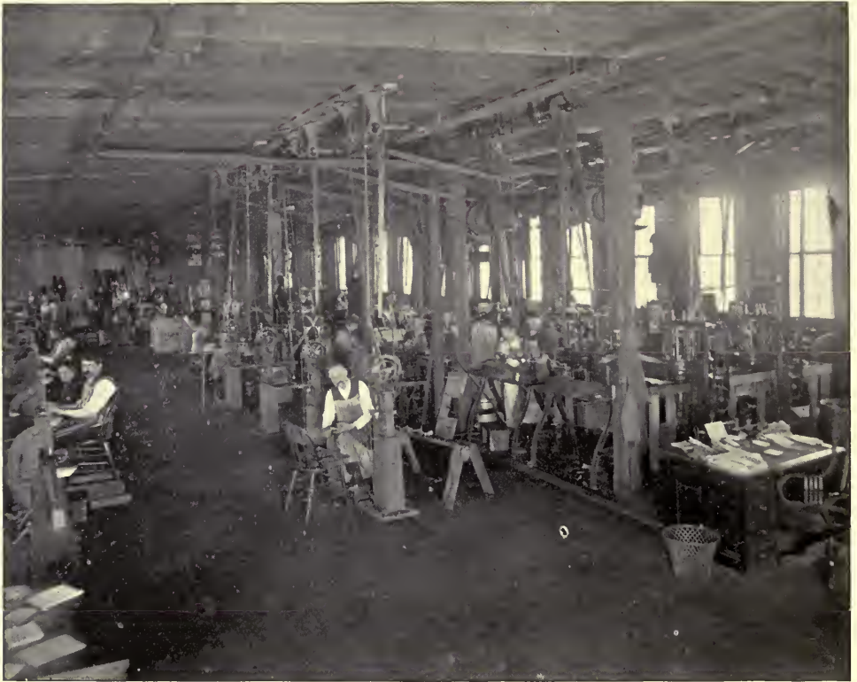
VIEW OF CHAIN AND PEDAL ROOM, BICYCLE DEPARTMENT. NATIONAL SEWING MACHINE CO.
