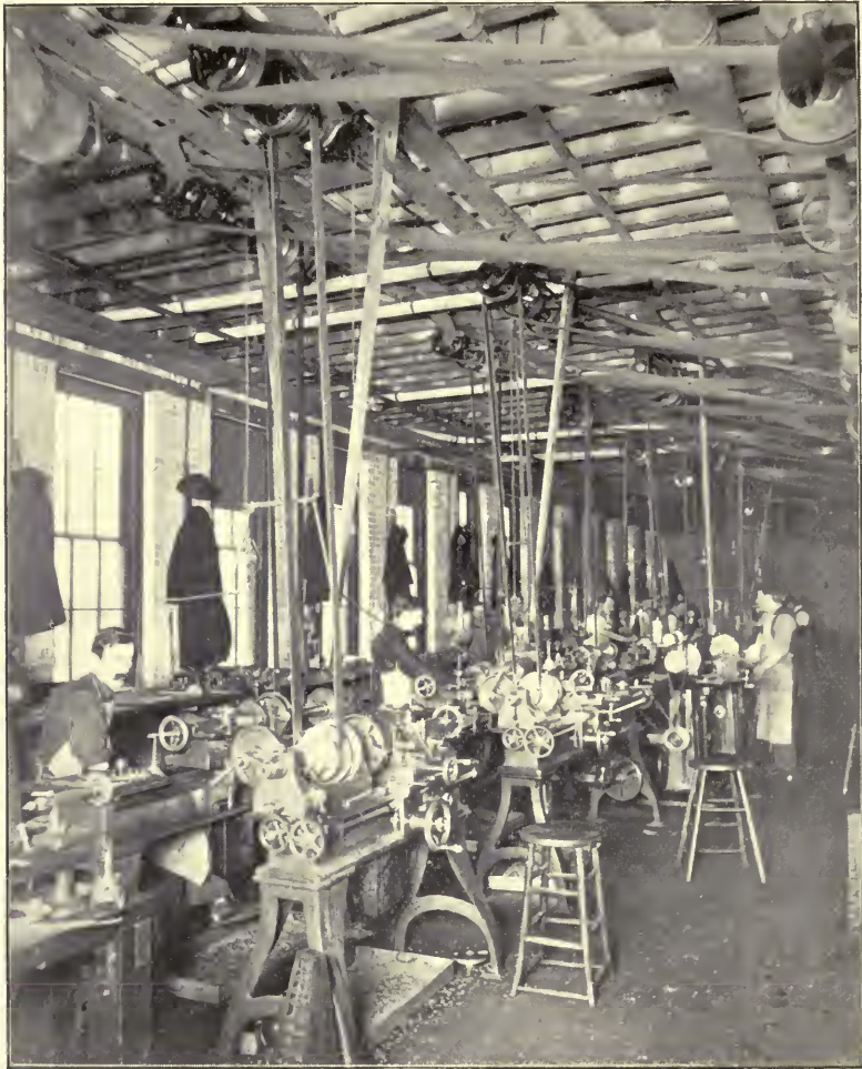
A GLIMPSE, OF THE TOOL ROOM, WESTERN AISLE.
