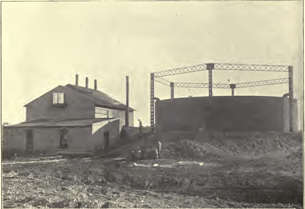
THE BELVIDERE GAS WORKS.
