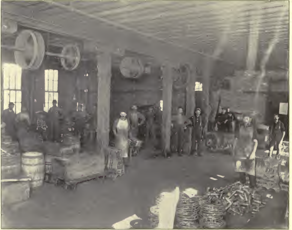
A GLANCE INTO THE GRINDING ROOM.
