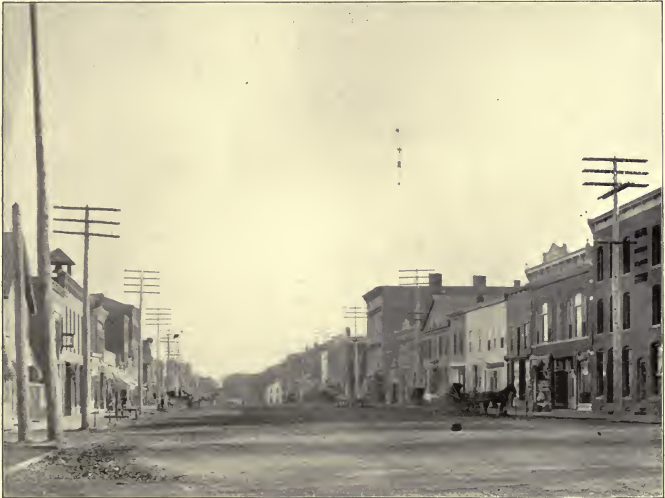
BUSINESS PORTION OF NORTH STATE STREET.
