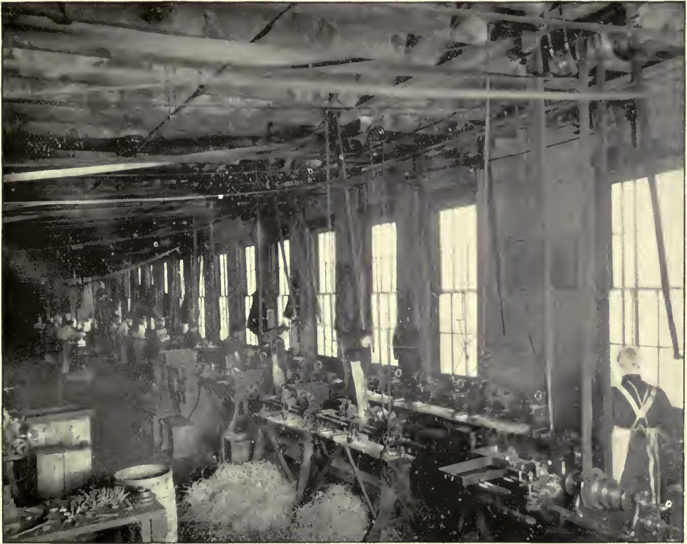
NORTH QUARTER OF LATHE ROOM.
