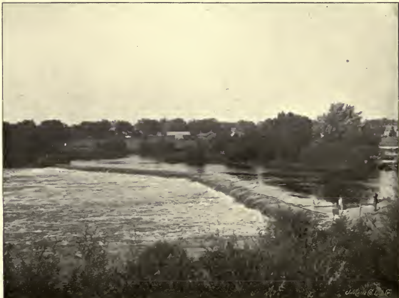
THE DAM BELOW THE CITY.
