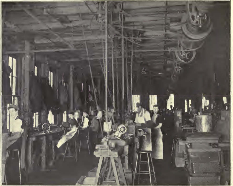
NORTH-WEST QUARTER OF SEWING MACHINE ASSEMBLING ROOM.
