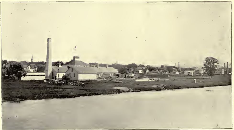
VIEW OF MILK CONDENSING FACTORY FROM RAILROAD BRIDGE. PHOTO BY CLARK & NOTT.
