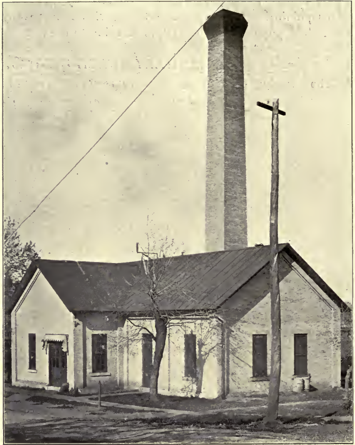
WATER WORKS BUILDING.
